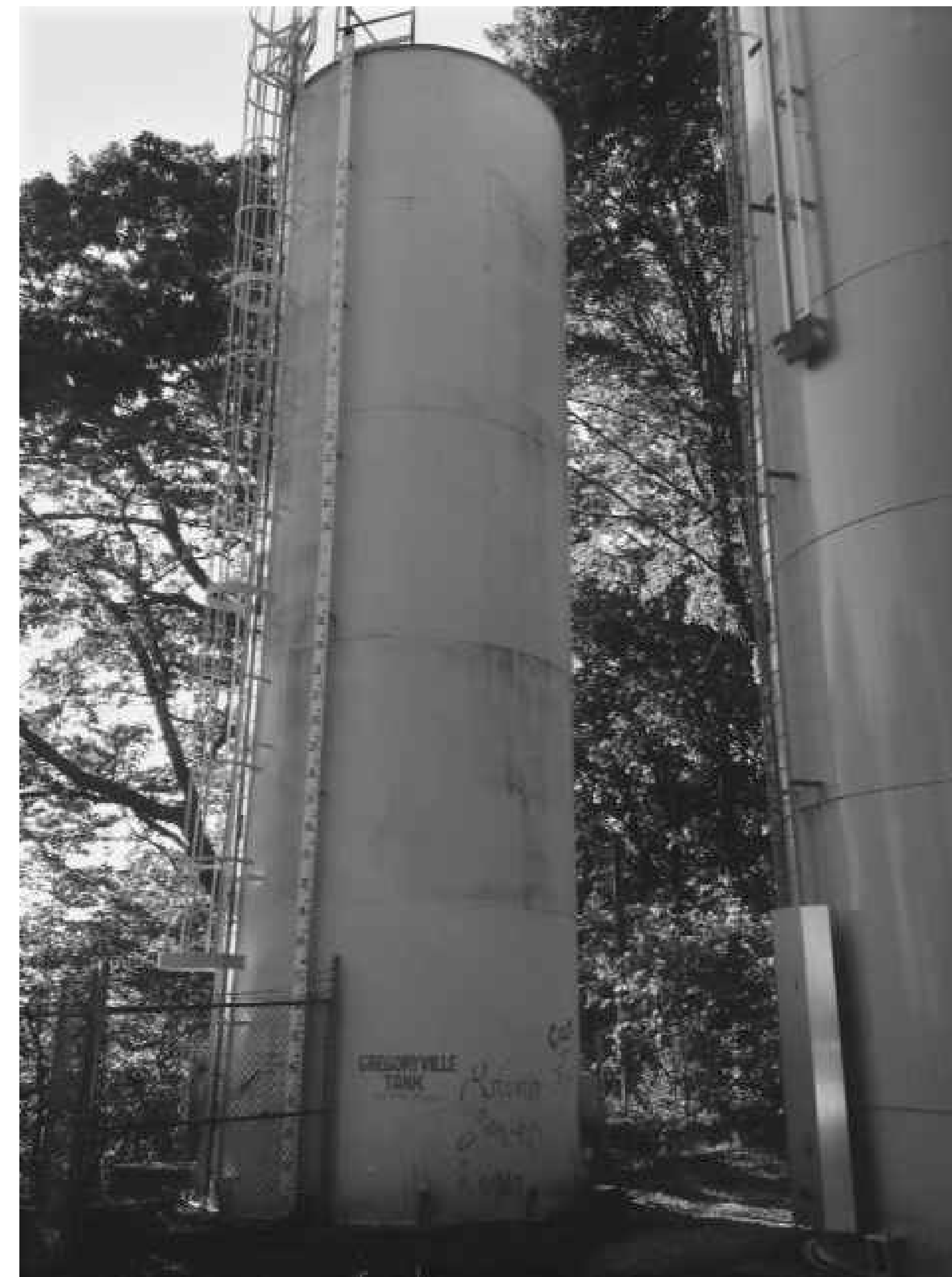
GROUND VIEW - GREGORYVILLE TANK #2
