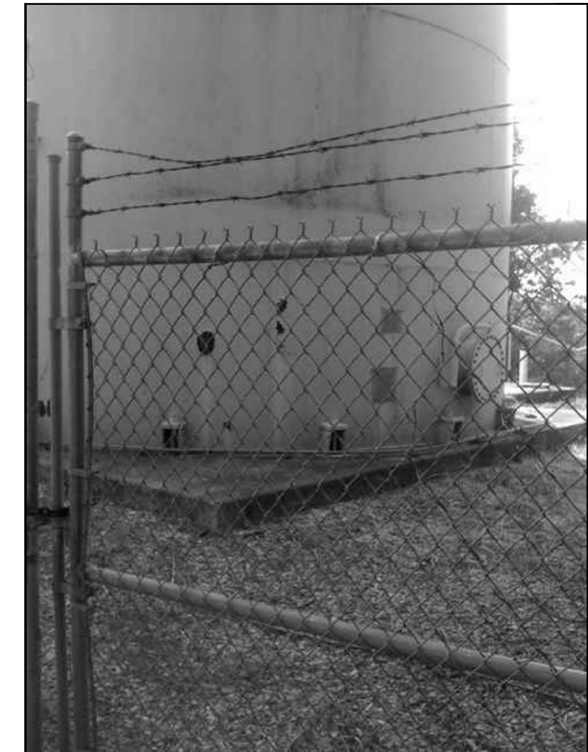
GROUND VIEW - FRANK JOHNSON TANK NOT TO SCALE
