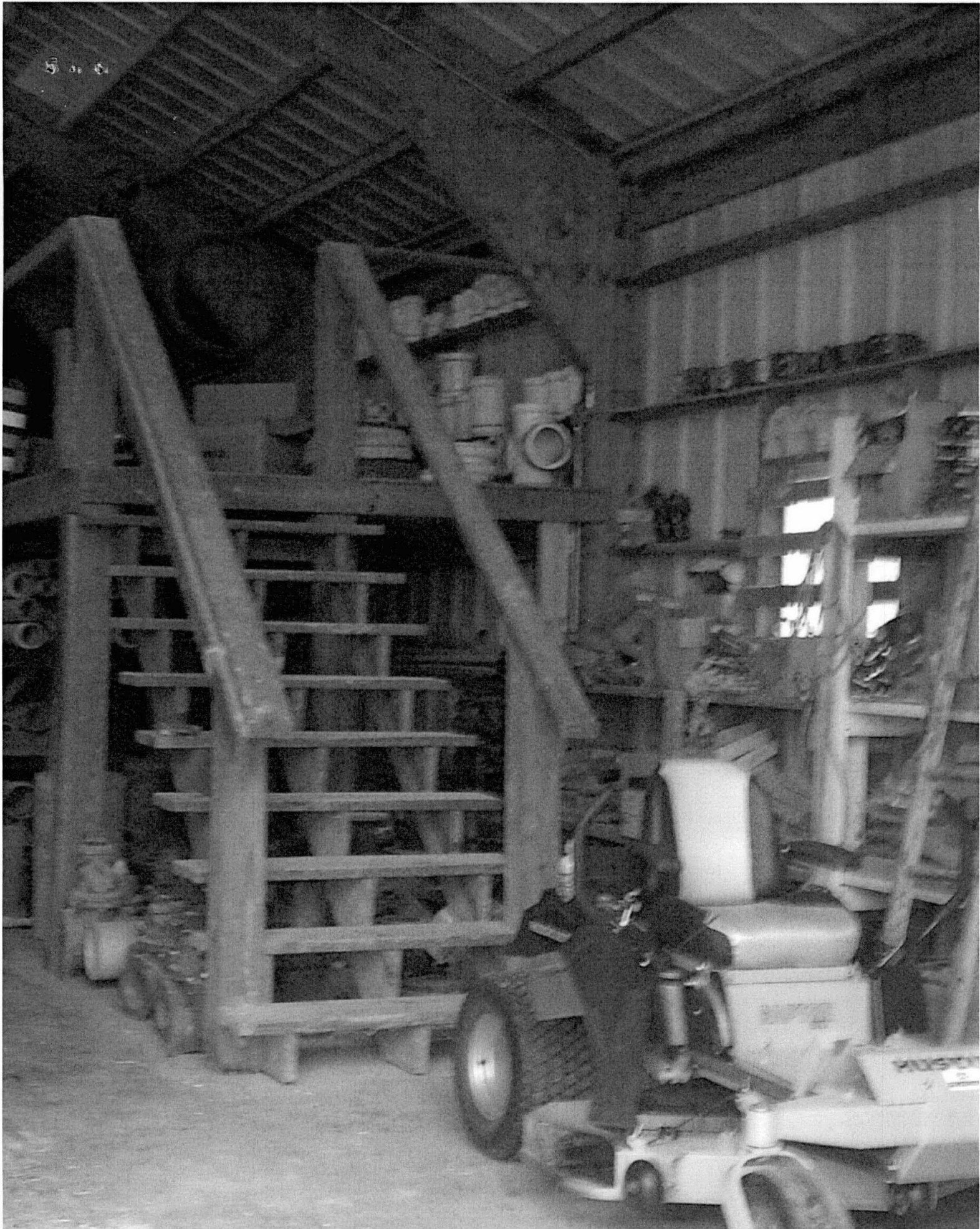
108 Main St. - Detached Metal Bldg
