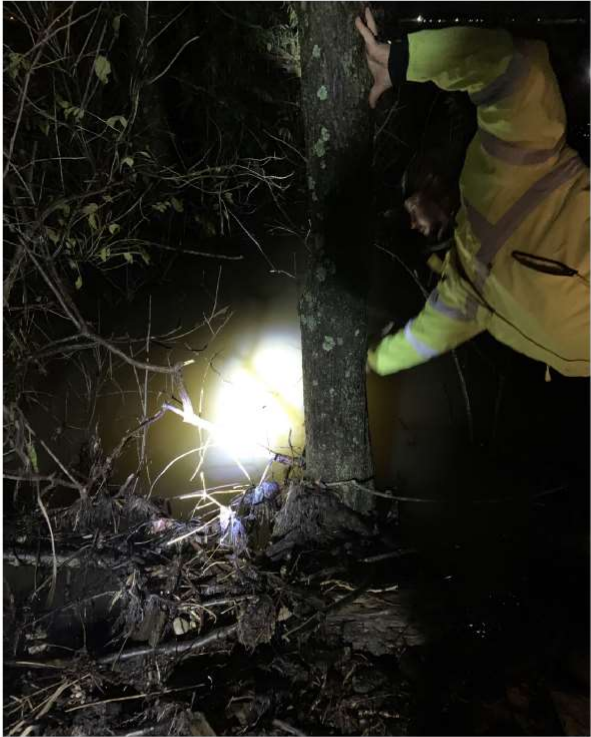
Approximate location of the damage.
