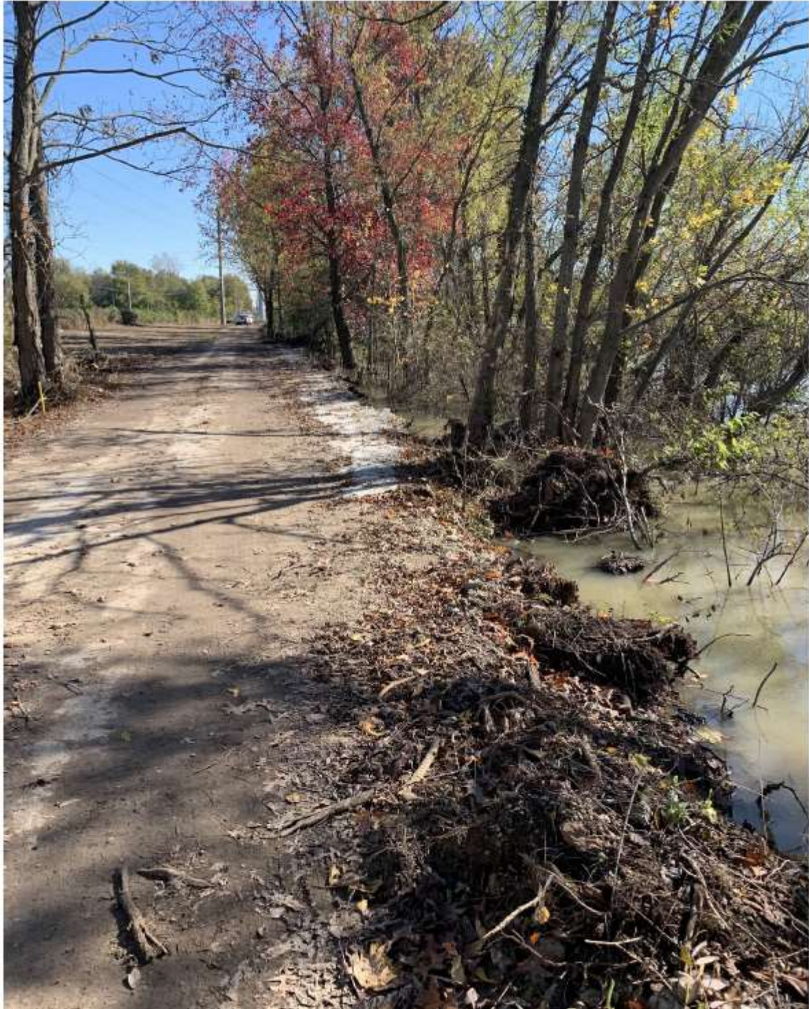
Area behind location of damage.
