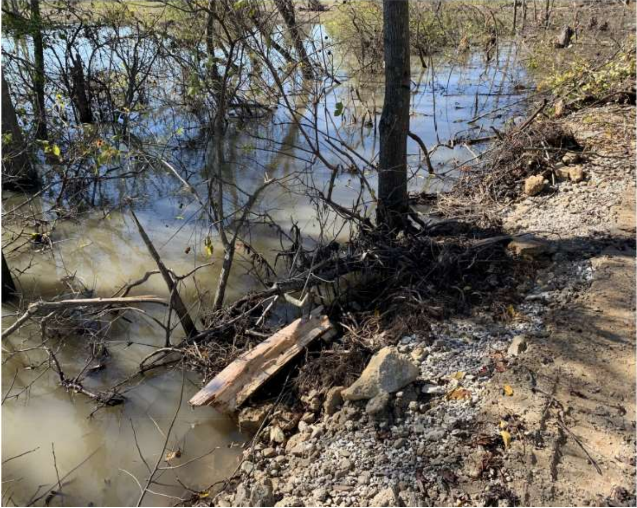
Approximate location of the damage.
