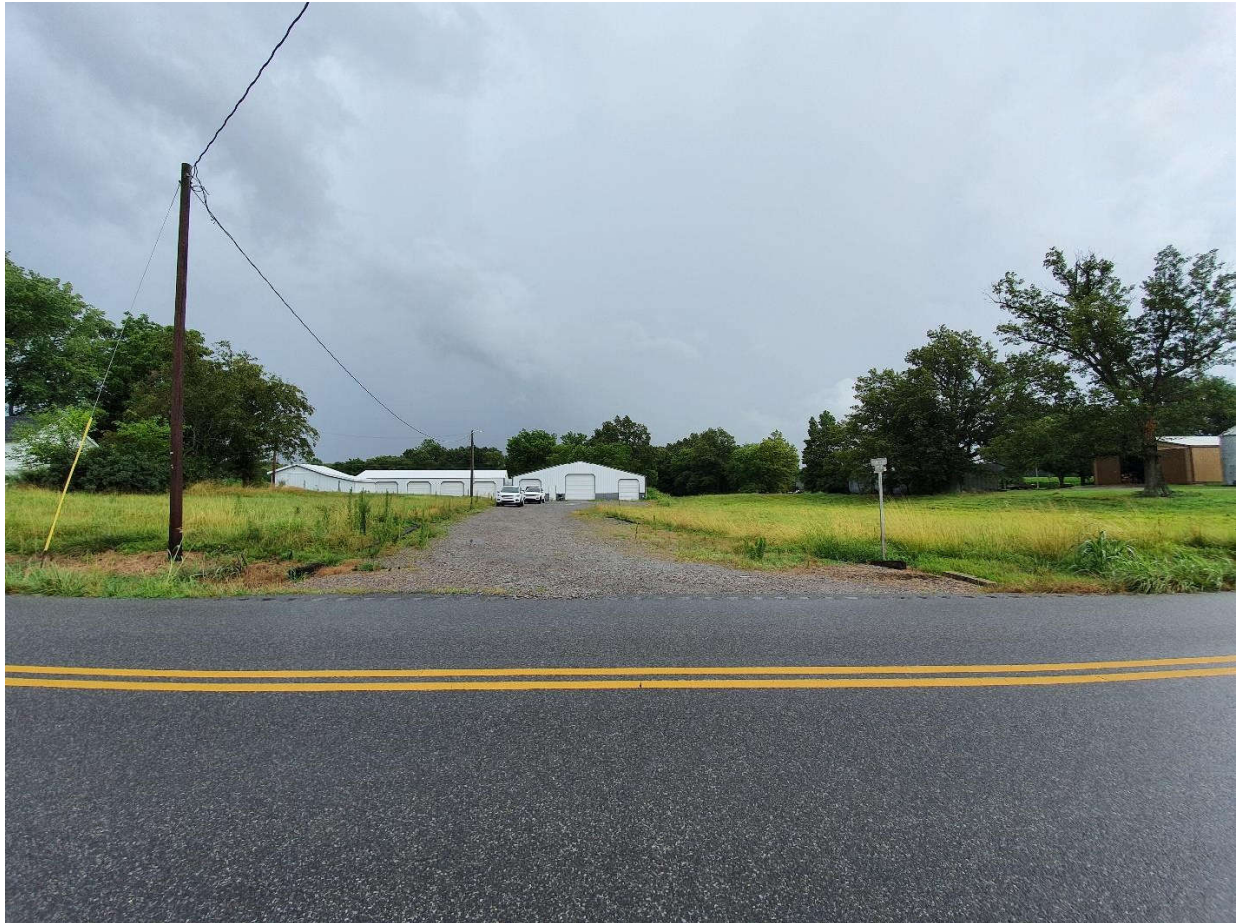
Picture (7) Location #6 – Substation Road Access
