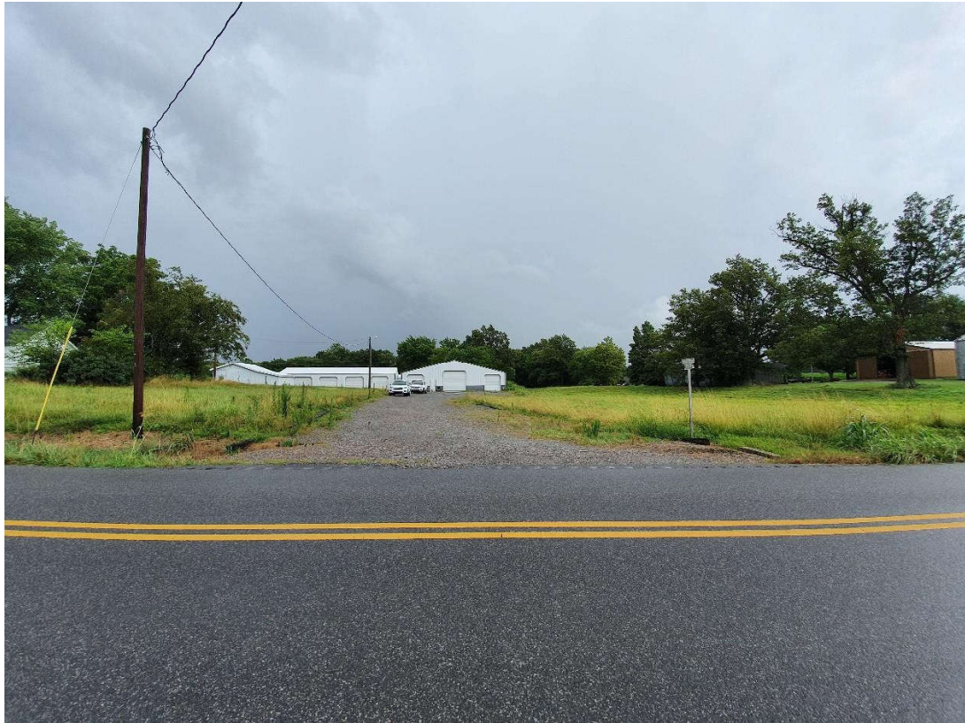
Picture (13) Existing Power Service Line
