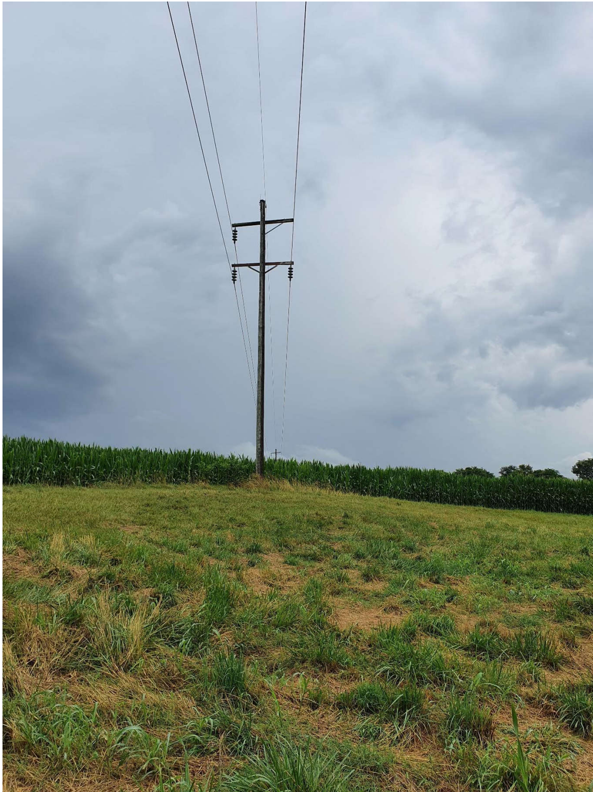
Picture (12) Location #7 – Big Rivers 69kV Interconnection
