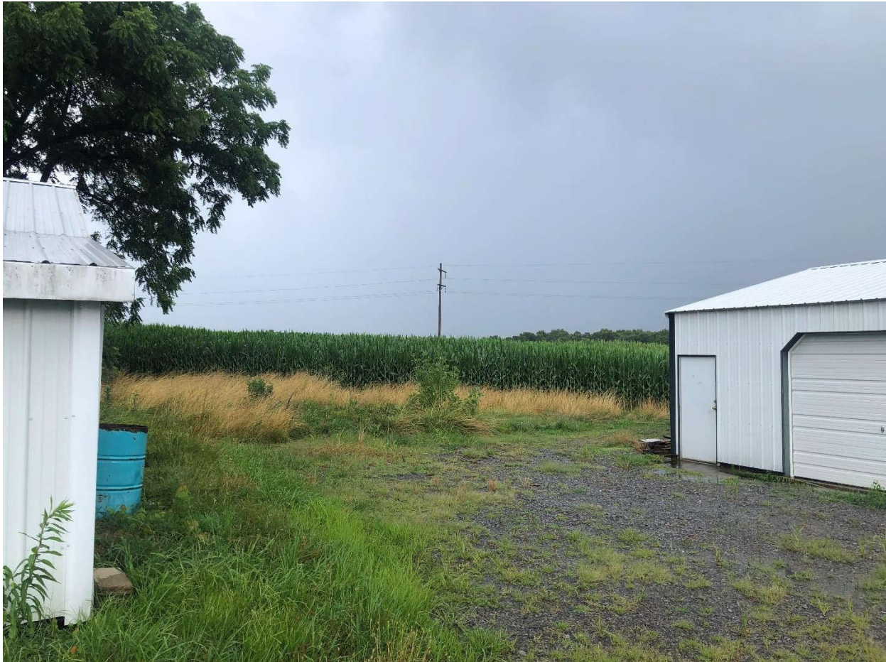
Picture (8) Location #6 – Big Rivers 69kV Line
