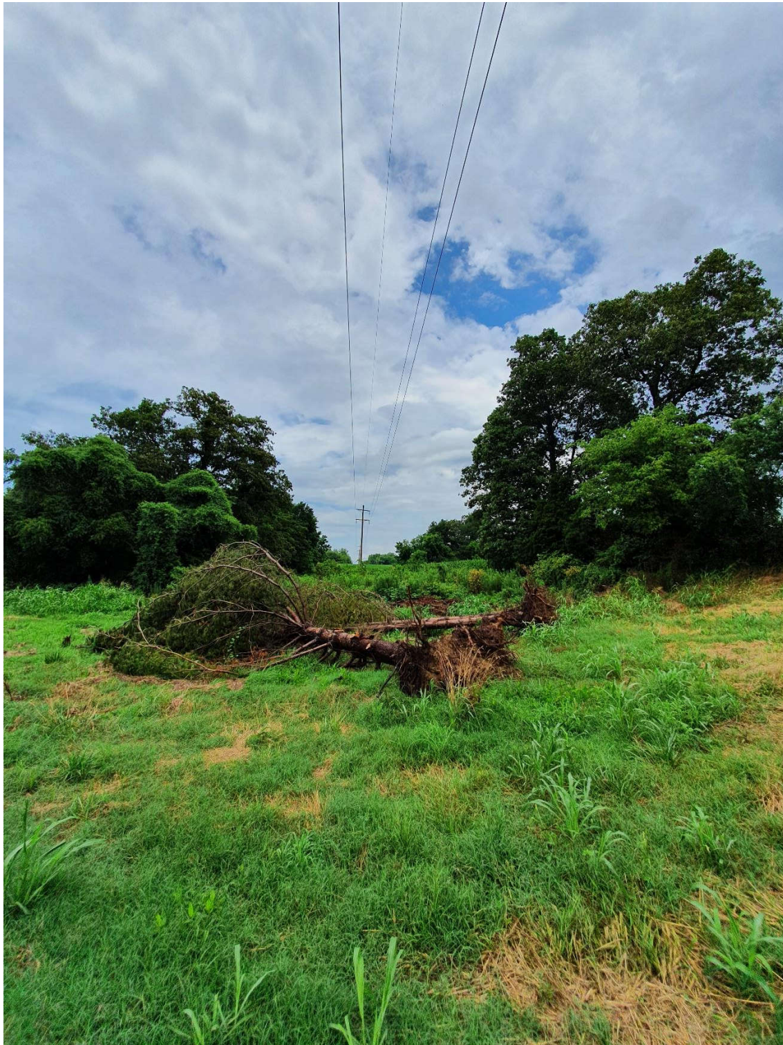
Picture (11) Location #7 – Big Rivers 69kV Interconnection
