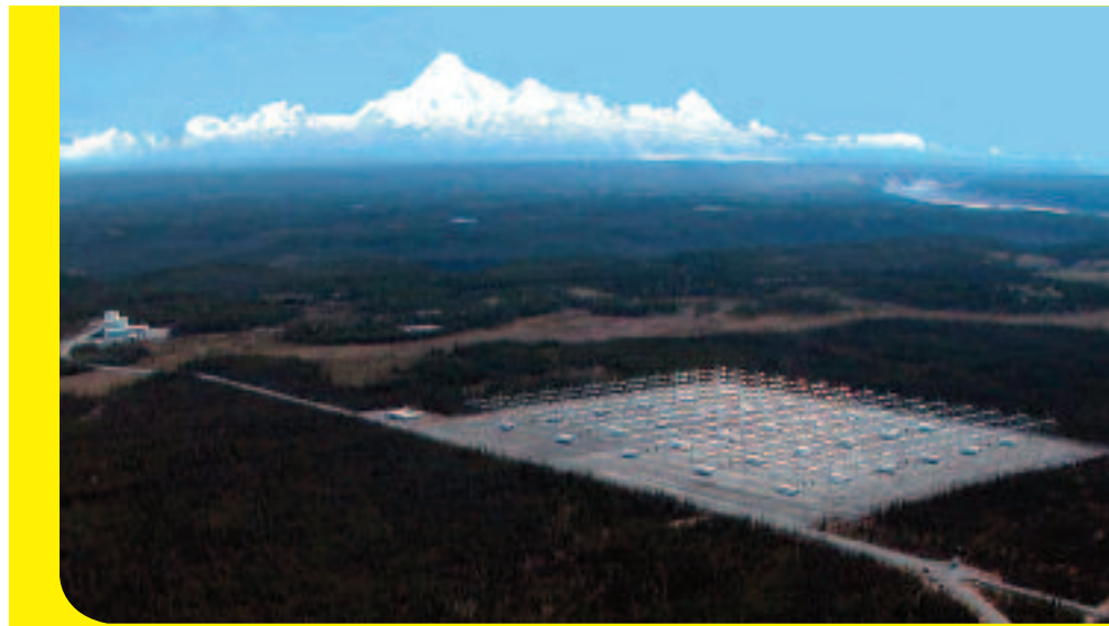
Fig. 25: HAARP location and construction.
