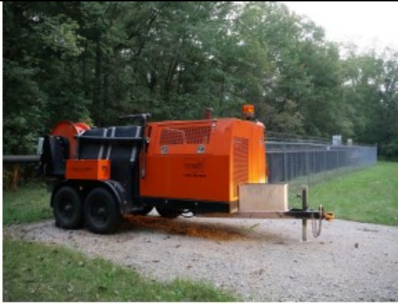
Backup generator on site for emergency power.
