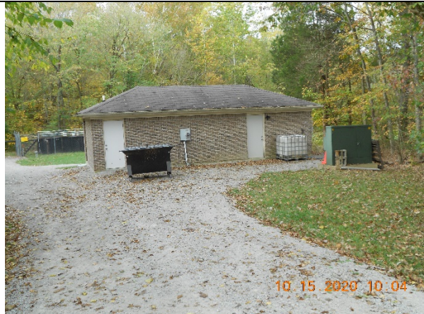
No repairs to blower house needed
