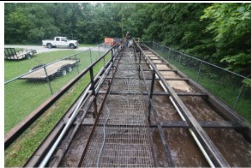
Damaged walkway sections replaced to ensure safety
