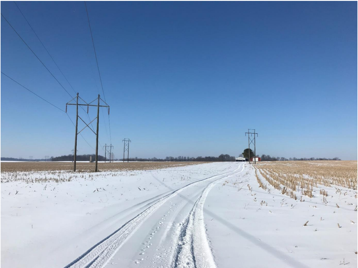
Figure C-5. View West from the Site of Potential Substation Location Near East Boundary of Site.
