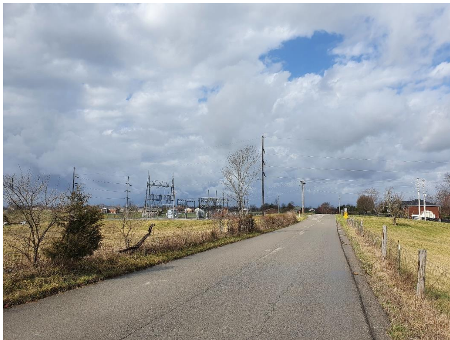
Picture (6) Location #5 – Existing Utility Substation
