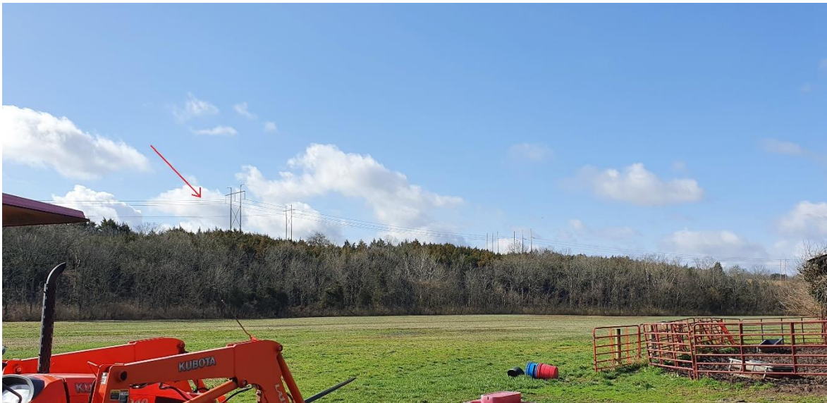
Picture (9) Power Lines
