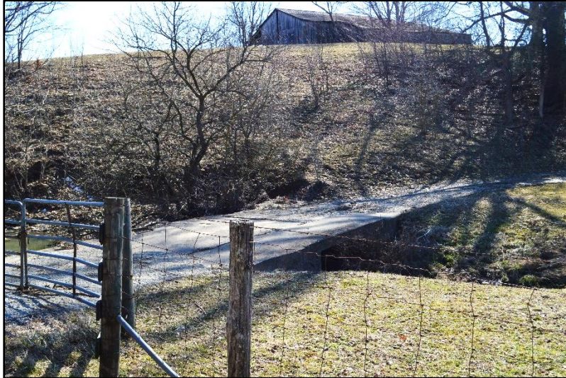
Figure B-29. Location of bridge near AP #7, facing southeast
