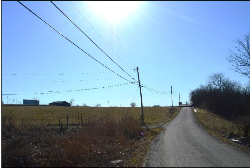
Figure B-3. Location near primary Access Point (AP) #2, facing southeast
