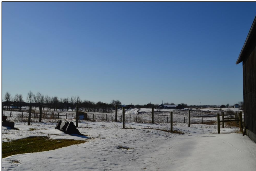
Figure B-20. Location near proposed substation, facing south/southeast
