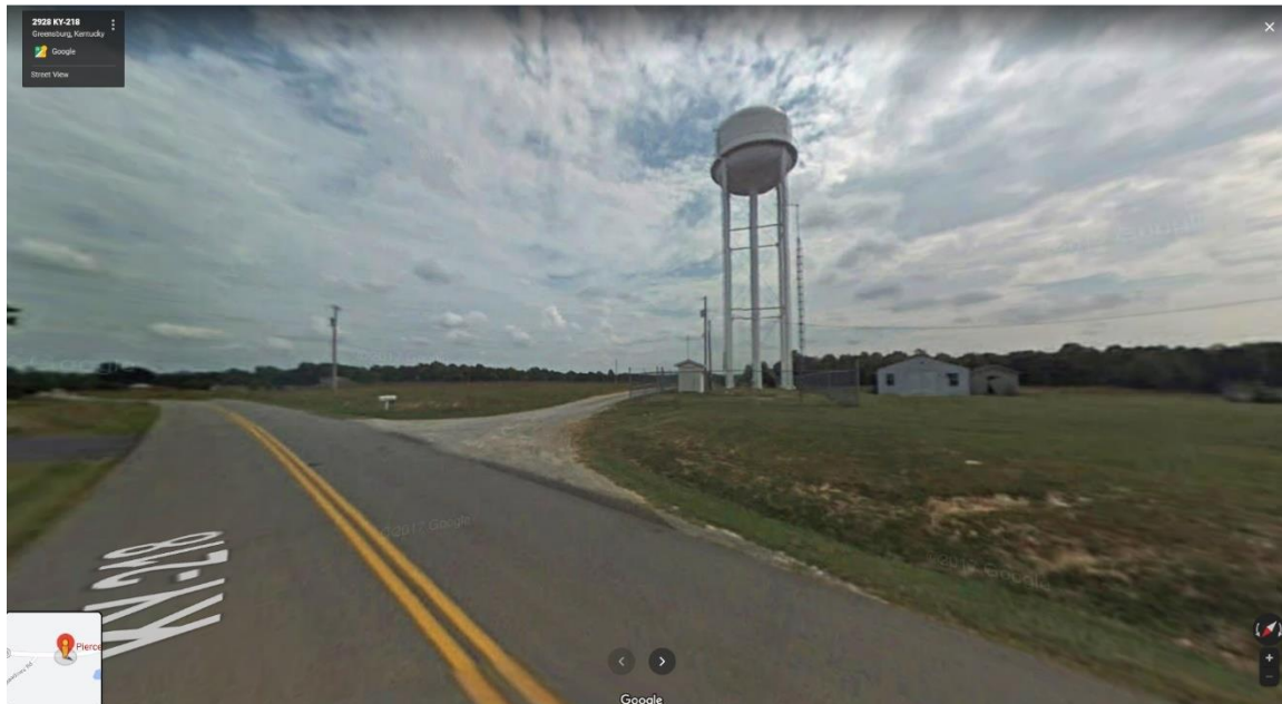
Picture (9) Overhead Tank on KY218 near Jim Meadows Road
