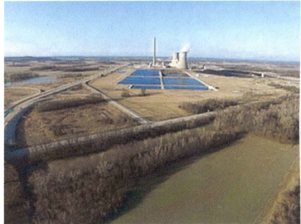
Rockport Generating Station as seen from near the Natcher Bridge
