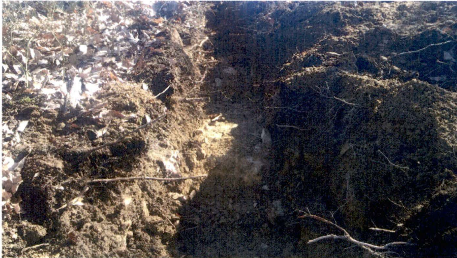
Sandstone Bottom of Trench
