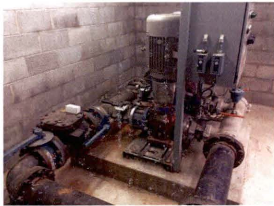
Eastern Pump Station
