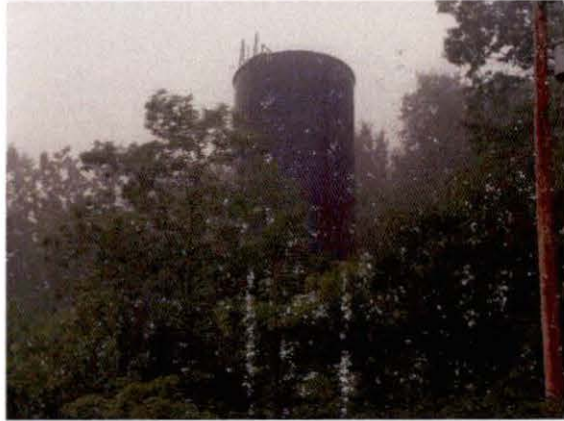
Spurlock Water Storage Tank
