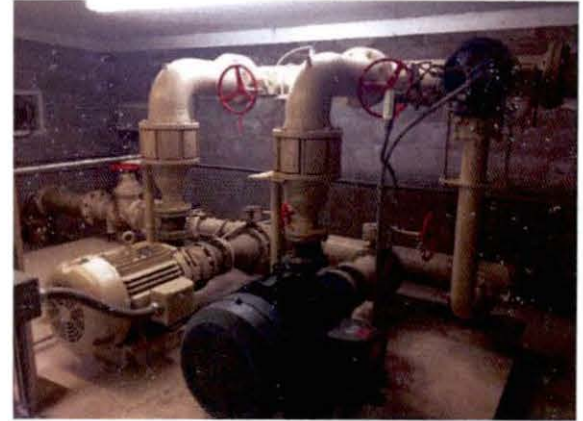
Fisher Hollow Pump Station
