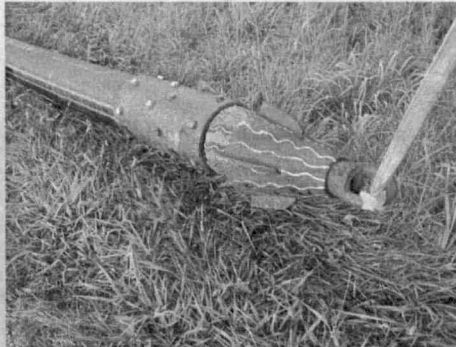
Pipe Splitting Apparatus
