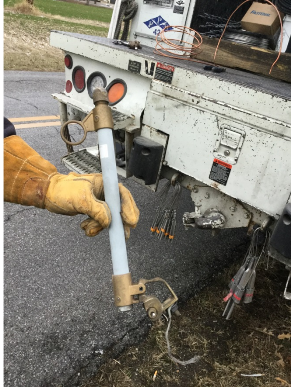
Pole_00008439 (Road Side Fuse - blown)
