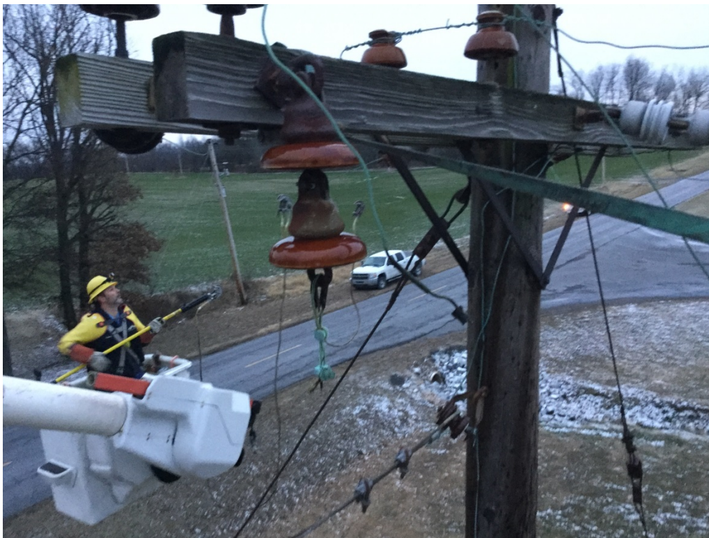
Pole_00008445 (Bells, 8A CWC deadend and Jumper over crossarm)
