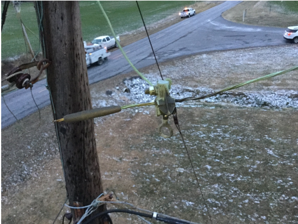
Pole_00008445 (8A CWC with Hotline Clamp to Phase running up Bethel Church Rd)
