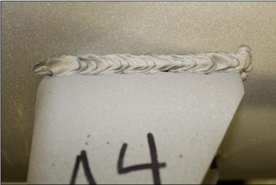
Figure 7. Image of the Lug A4 exterior bottom weld which exhibited substantial fusion.
