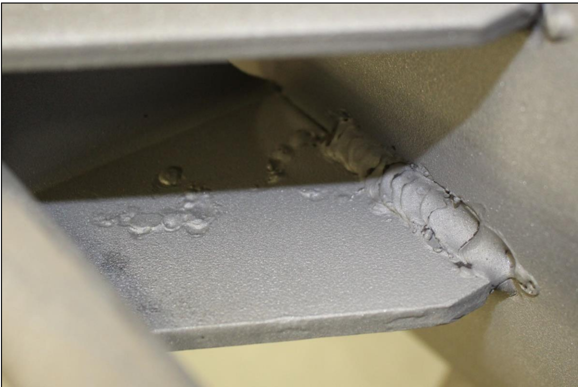
Figure 12. Image of the Lug B5 interior bottom weld which exhibited substantial fusion except for arc strikes, porosity, and spatter.
