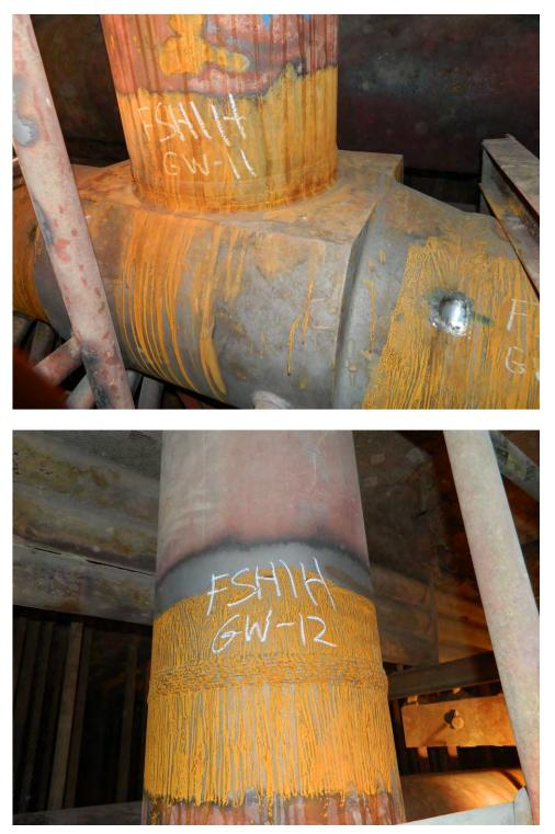
Fig. 38. Photographs of girth weld Nos.GW-11 and GW-12 on the Finishing Superheater Inlet header.
