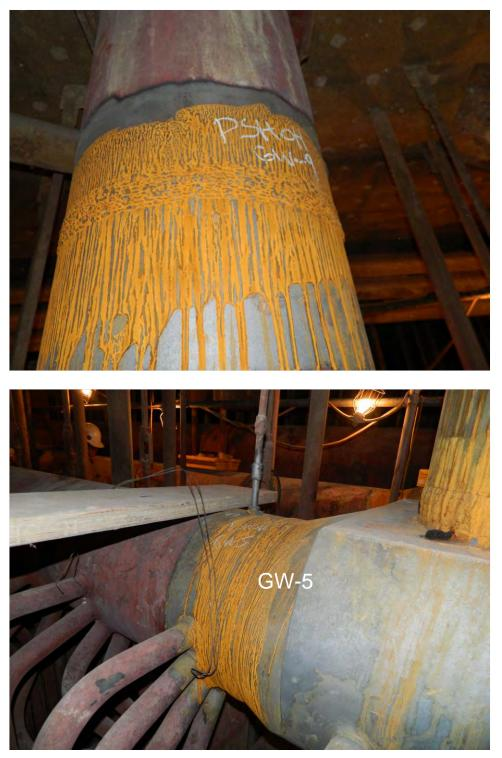
Fig. 18. Photographs of girth weld Nos. GW-4 and GW-5 on the Platen Superheater Outlet header.
