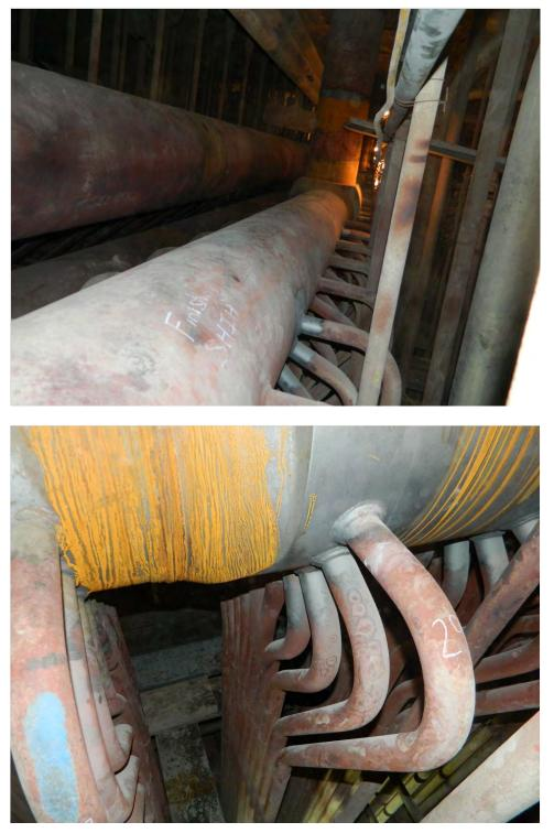
Fig. 32. Photographs of the Finishing Superheater Inlet header and tubing.
