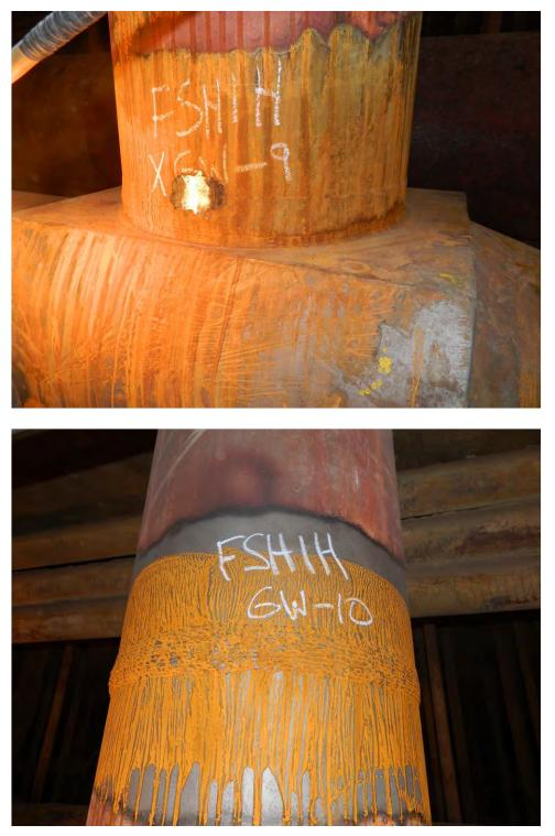
Fig. 37. Photographs of girth weld Nos.GW-9 and GW-10 on the Finishing Superheater Inlet header.
