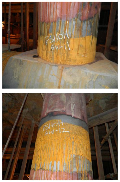
Fig. 21. Photographs of girth weld Nos. GW-11 and GW-12 on the Platen Superheater Outlet header
