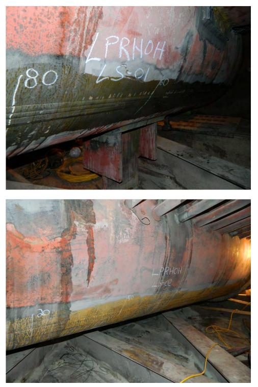
Fig. 88. Photographs of seam weld Nos.LS-01 and LS-02 on the LP Reheat Outlet header.
