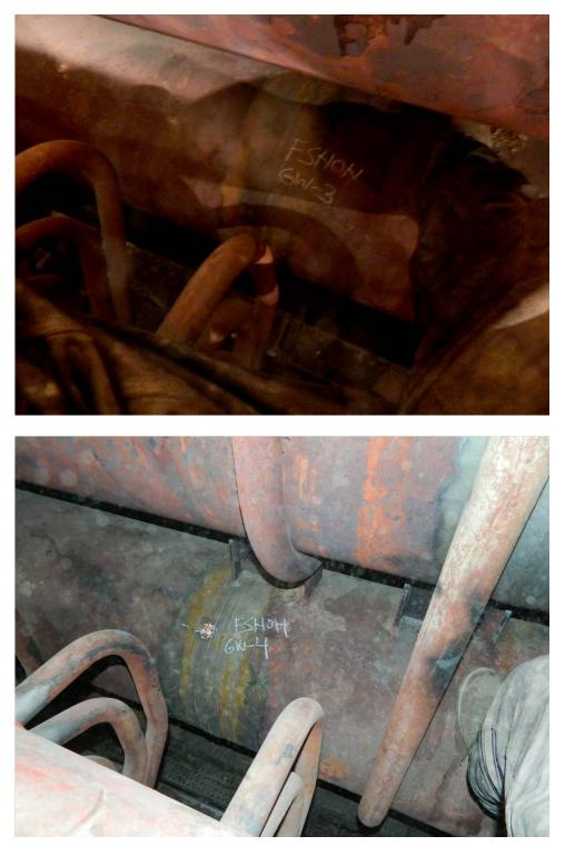
Fig. 54. Photographs of girth weld Nos. GW-3 and GW-4 on the Lower Finishing Superheater Outlet header.
