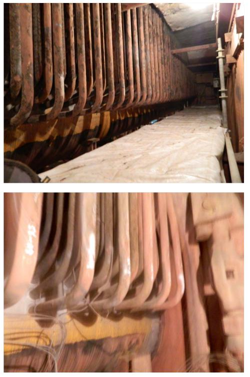
Fig. 73. Photographs of the HP Reheat Outlet header and tubing.
