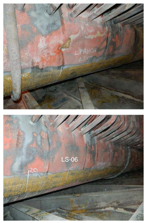
Fig. 89. Photographs of seam weld Nos.LS-04 and LS-06 on the LP Reheat Outlet header.
