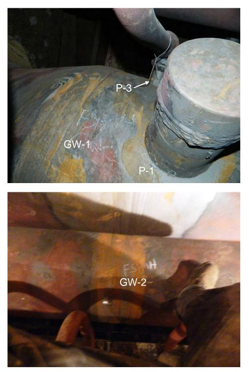
Fig. 53. Photographs of penetration Nos. P-1, P-2, and girth weld Nos. GW-1 and GW-2 on the Lower Finishing Superheater Outlet header.
