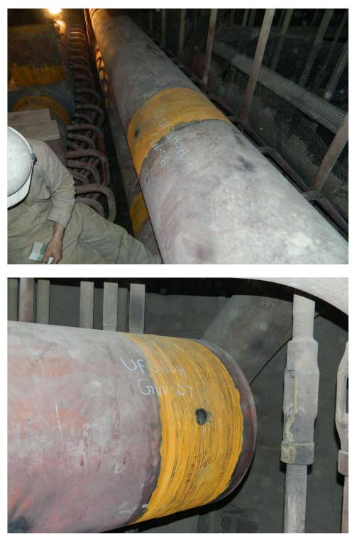
Fig. 52. Photographs of girth weld Nos. GW-6 and GW-7 on the Upper Finishing Superheater Outlet header.
