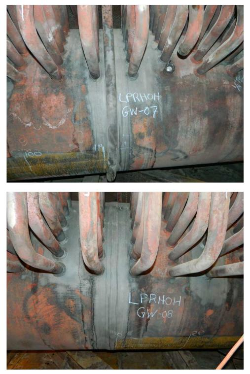
Fig. 87. Photographs of girth weld Nos. GW-7 and GW-8 on the LP Reheat Outlet header.
