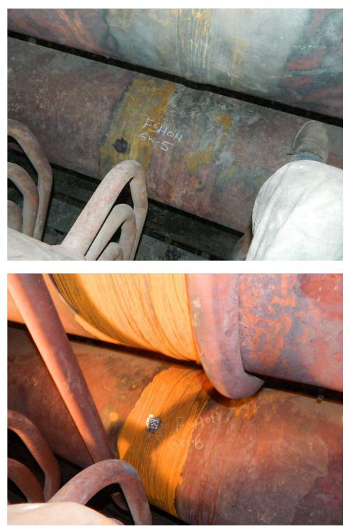
Fig. 55. Photographs of girth weld Nos. GW-5 and GW-6 on the Lower Finishing Superheater Outlet header.
