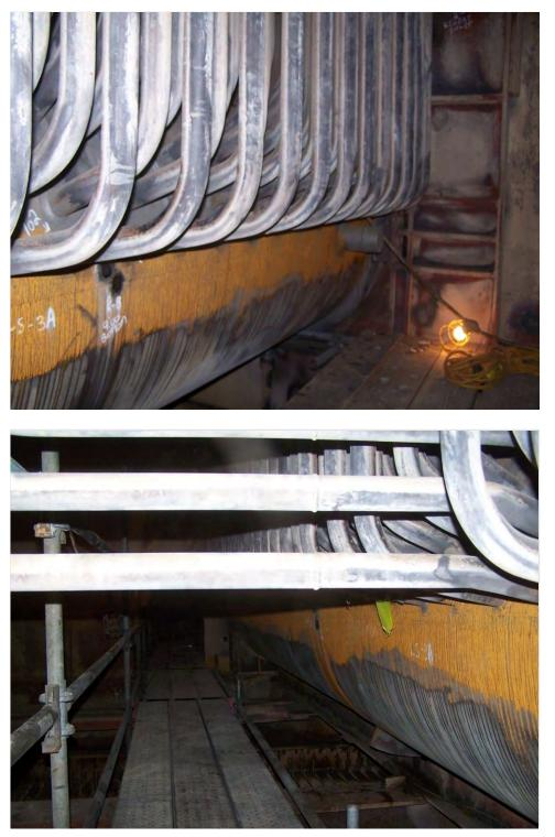
Fig. 136. Photographs of the inspection locations on the Low-Pressure (2nd) Reheat Inlet header and tube stubs.
