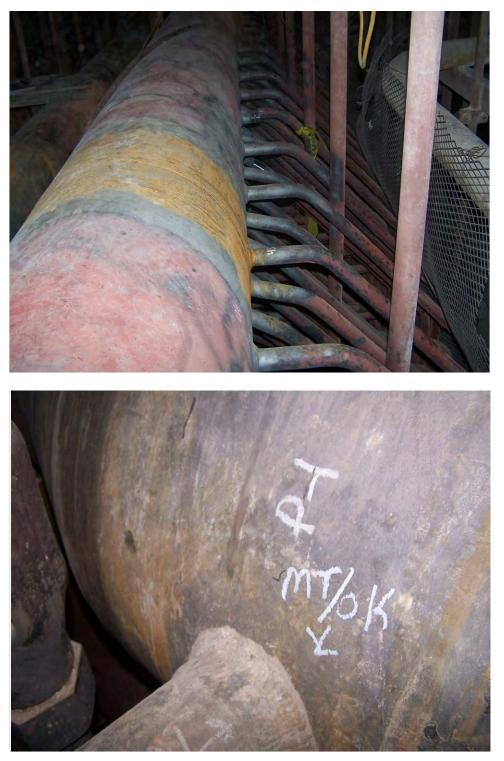
Fig. 48. Photographs of the inspection locations on the Upper Finishing Superheater Outlet header.
