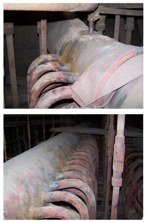
Fig. 2. Photographs of the Platen Superheater Inlet header and tubing.
