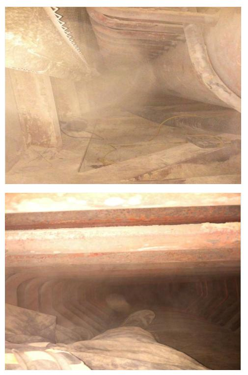
Fig. 113. Photographs of the inspection locations on the Low-Pressure Reheat Outlet header and tube stubs.
