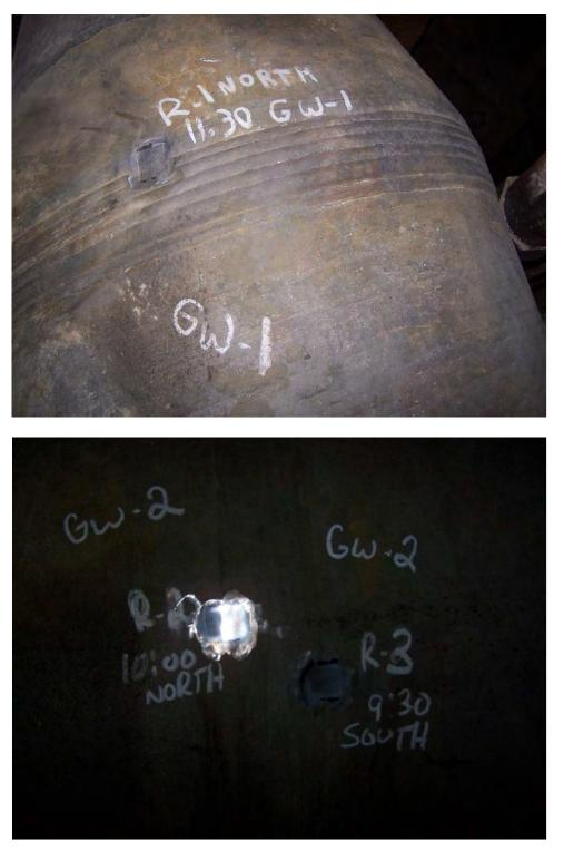
Fig. 49. Photographs of the inspection locations on the Upper Finishing Superheater Outlet header.
