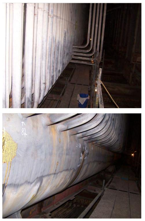
Fig. 124. Photographs of the inspection locations on the High-Pressure (1st) Reheat Inlet header and tube stubs.
