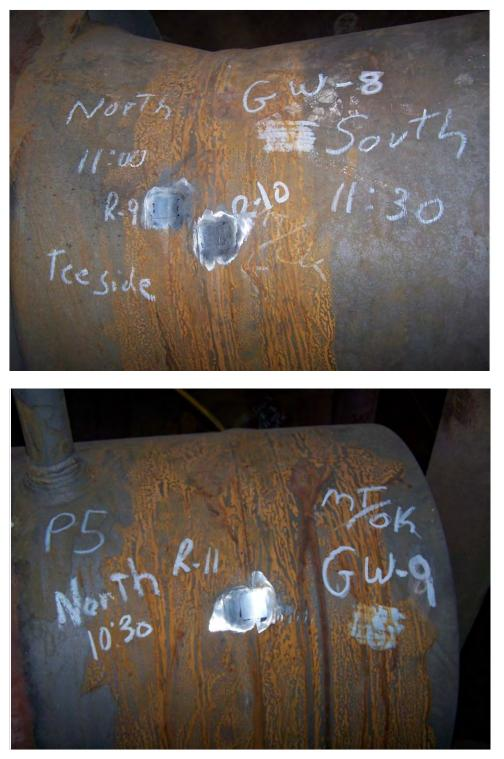
Fig. 33. Photographs of the inspection locations on the Finishing Superheater Inlet header.
