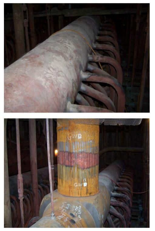
Fig. 14. Photographs of the inspection locations on the Platen Superheater Outlet header.
