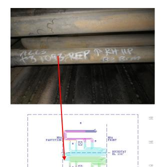
HIGH PRESSURE REHEATER INLET SECTION
