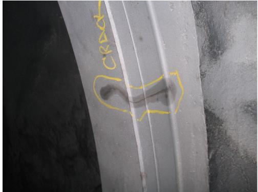
Mid-span Ecc Hole Crack
