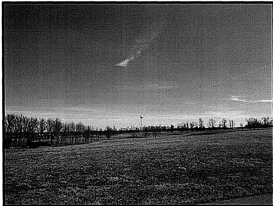
View of 50KG Tank From Eagle Drive
