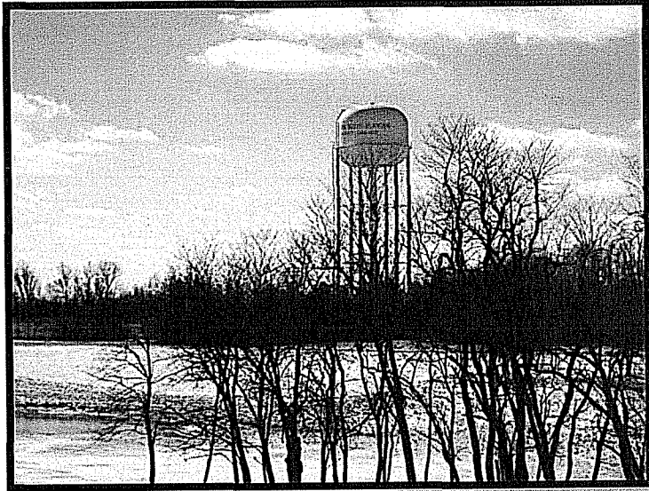
View of 500KG tank Behind 302 Eagle Drive
