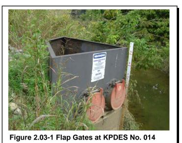
station. In April 2008, HWU sealed the flap gates resulting in zero overflows in the four and a half months since (from mid-April through the end of August). In the three months prior to sealing the flap gates, this pumping station had an overflow volume of 86 million gallons. The improvement at the pumping station has resulted in a significant improvement in the CSS. Figure 2.03-1 is a picture of the two flap gates at the Second Street Pumping Station.
