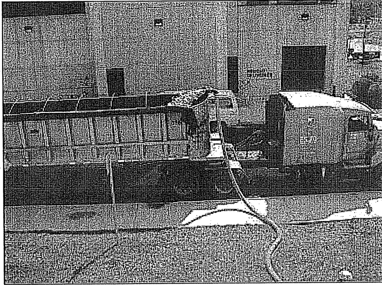
EXHIBIT 5-29 Media Removal by Eduction to Open-Bed Truck (Provided by Calgon Carbon Corporation)
