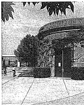
The Bingham Way Flood Pumping Station, which is located next to Riverfront Park, protects portions of downtown Louisville Metro.
