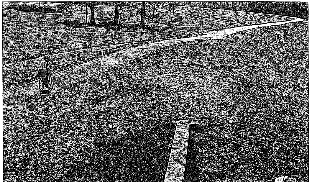
The Ohio River Levee Trail offers access and recreational opportunities along the Ohio River.
