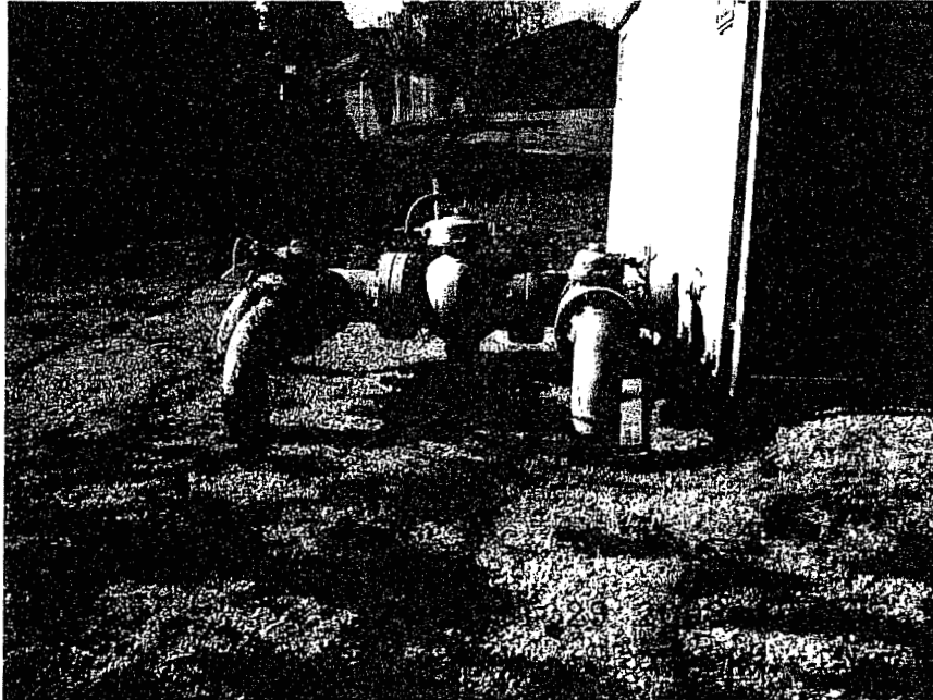
Valve for Incoming Line at City Gate Station
