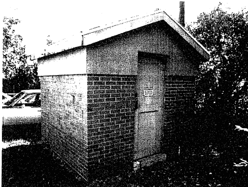
Oakland Drive Regulating Station
