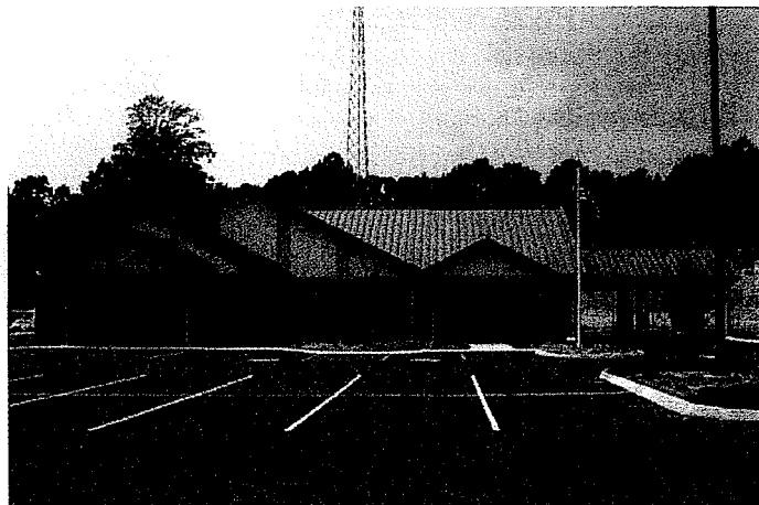
The new Whitley City office was completed in August 2006. All the new South Kentucky RECC district offices will be the same floor plan and size.
