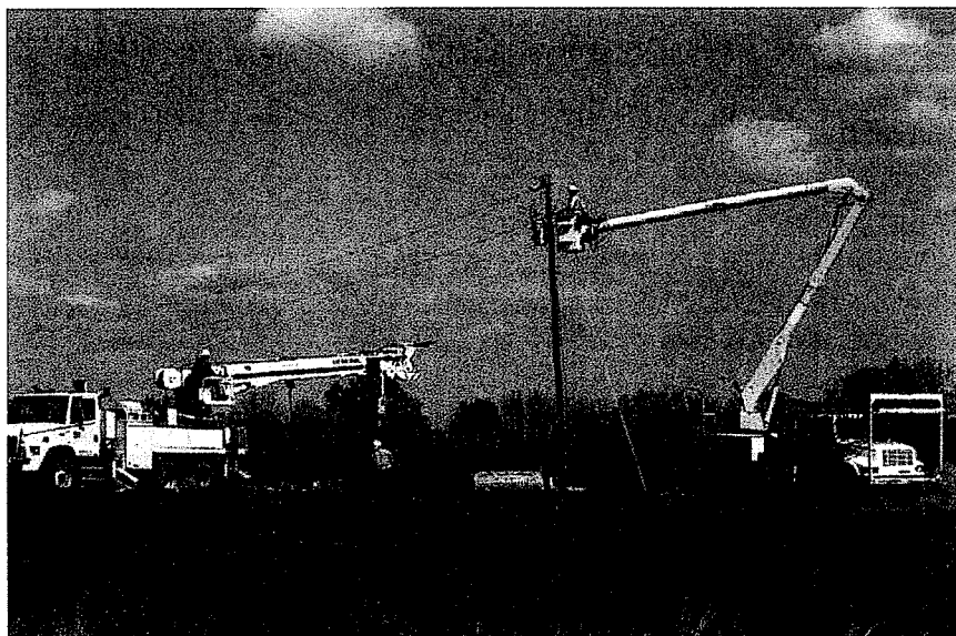
A large portion of South Kentucky RECC's new work plan is for new service extensions. Here, an SKRECC construction crew begins setting poles and establishing service in a new Wayne County subdivision.
