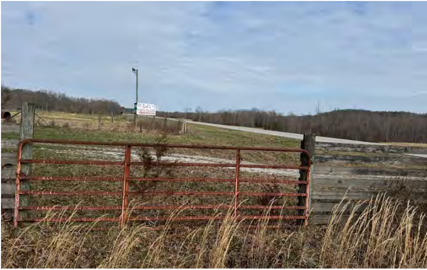
I: Westerly View of Existing Access Road from the Proposed Access/Utility Easement
