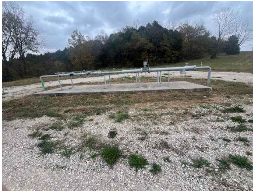
PHOTO 2: PHOTO OF THE NEW REGULATOR STATION INSTALLED IN 2015 AT THE NORTHWEST CORNER OF THE SERVICE AREA.
