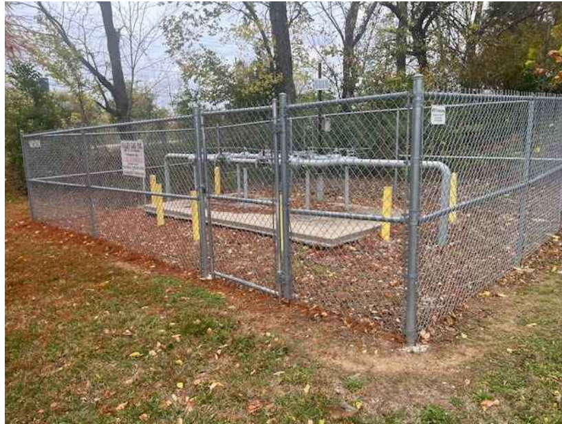
PHOTO 2: PHOTO OF THE NEW REGULATOR STATION INSTALLED IN 2015 AT THE NORTHWEST CORNER OF THE SERVICE AREA.
