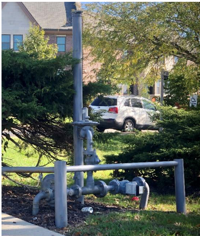
Relief Valve Assembly
