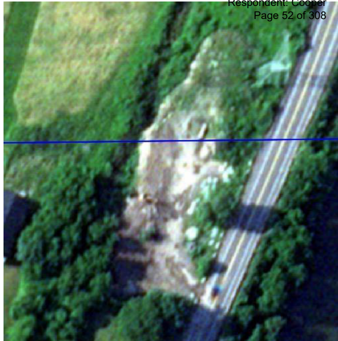
Image showing new excavation activity.
