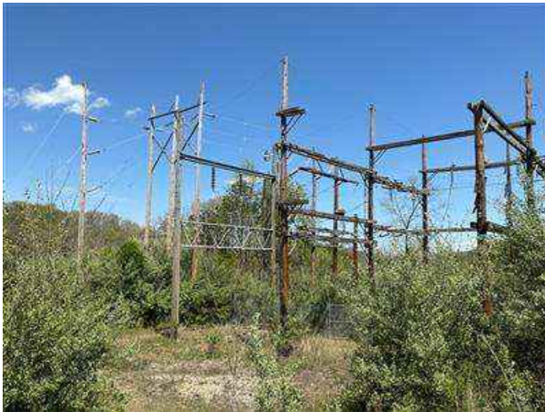
View of an abandoned/decommissioned electrical substation on the eastern portion of the Subject Property (Pocahontas parcel 040-00-00-020.00).
