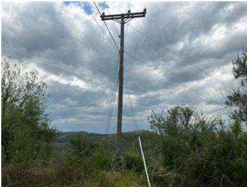
Overview of an electrical transmission line corridor.
