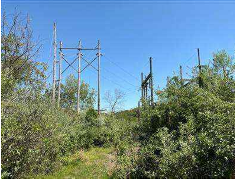
View of an abandoned/decommissioned electrical substation on the eastern portion of the Subject Property (Pocahontas parcel 040-00-00-020.00).
