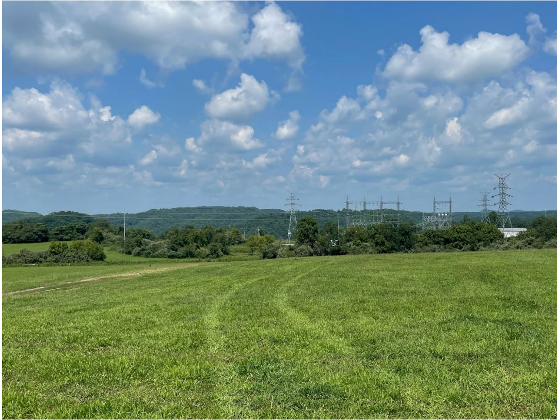
Figure C-7. Inez substation viewed from the site of the Martin County solar generating facility in 2021.
