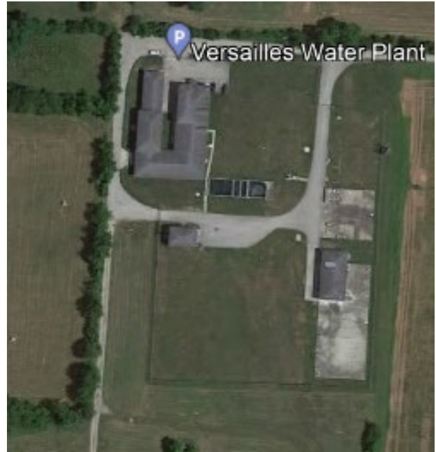
Figure 4-14 VMU WTP Site
