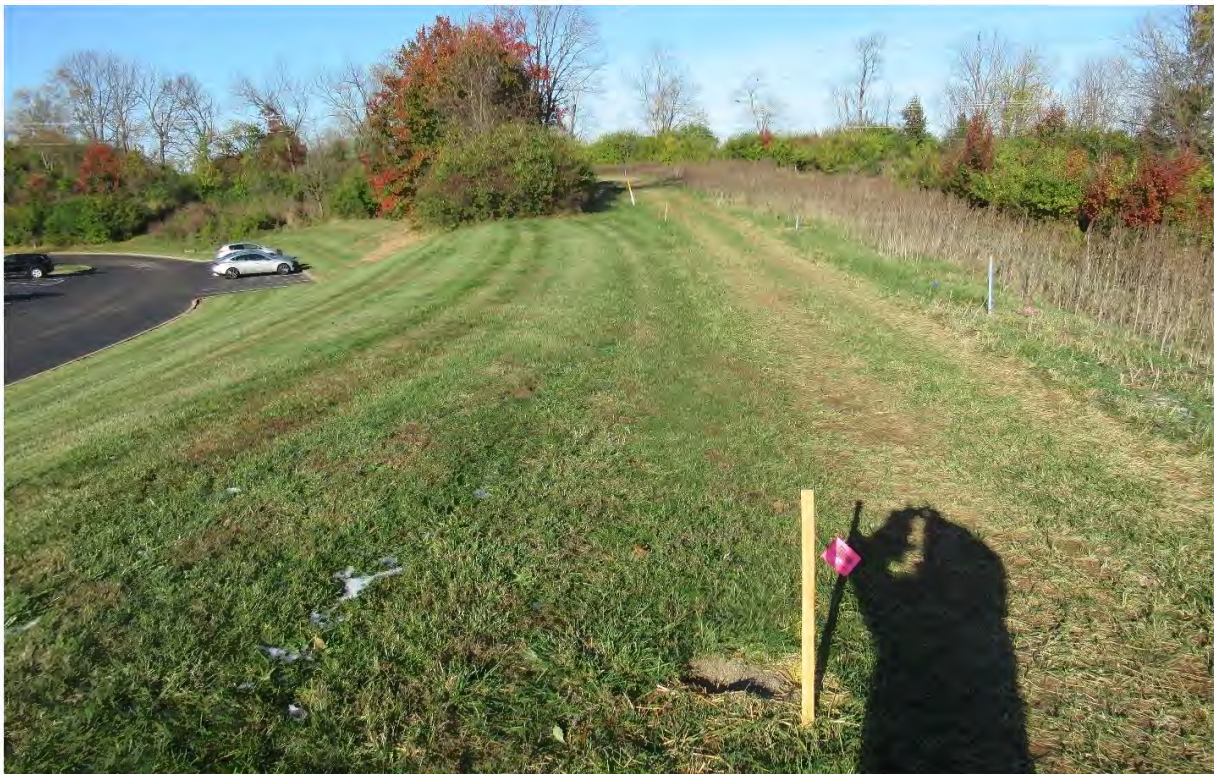
Figure 3: Main Corridor Near Apartment Complex
