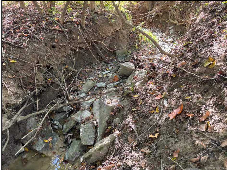
Photo 15: View upstream of intermittent S06, facing west.
