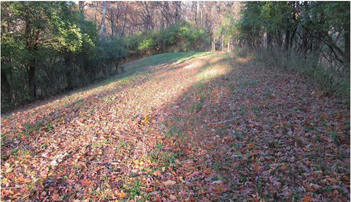
Figure 20: Existing Pipeline ROW on Ridge Crest
