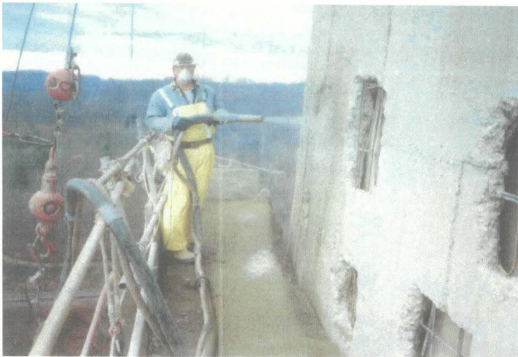
Shotcrete repair in progress
