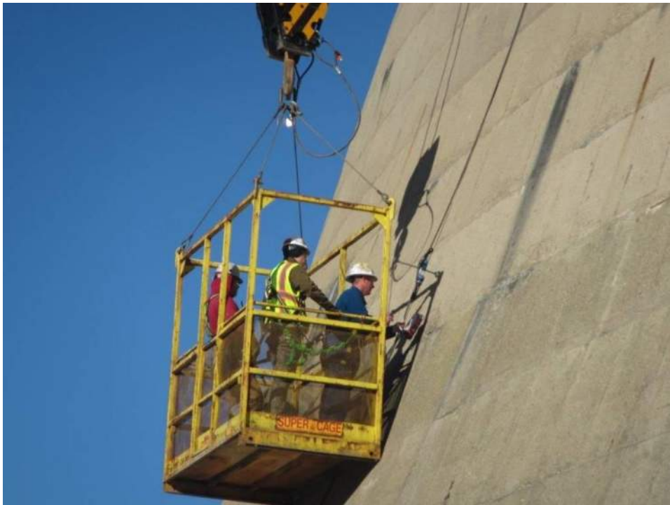
Photo 2. Visual review of the concrete veil
