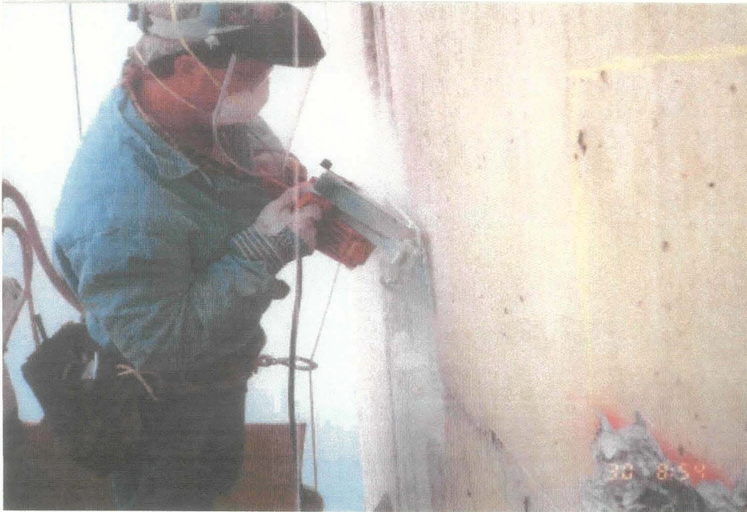
Saw-cutting around perimeter of repair areas
