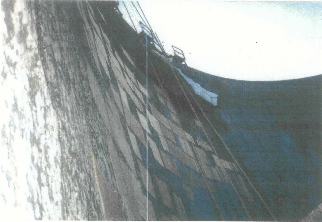
Forms on interior of shell
