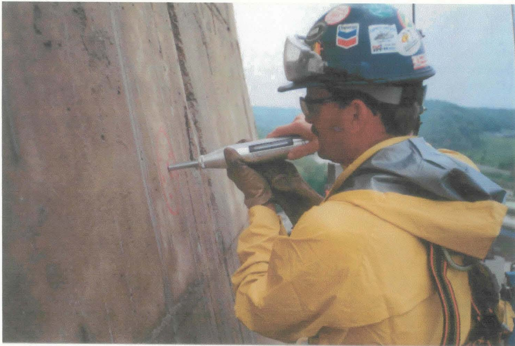
Specimen Photograph No. 13 Rebound hammer testing
