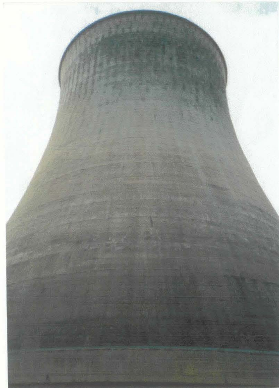
Site Photograph No. 4 Southeast elevation
