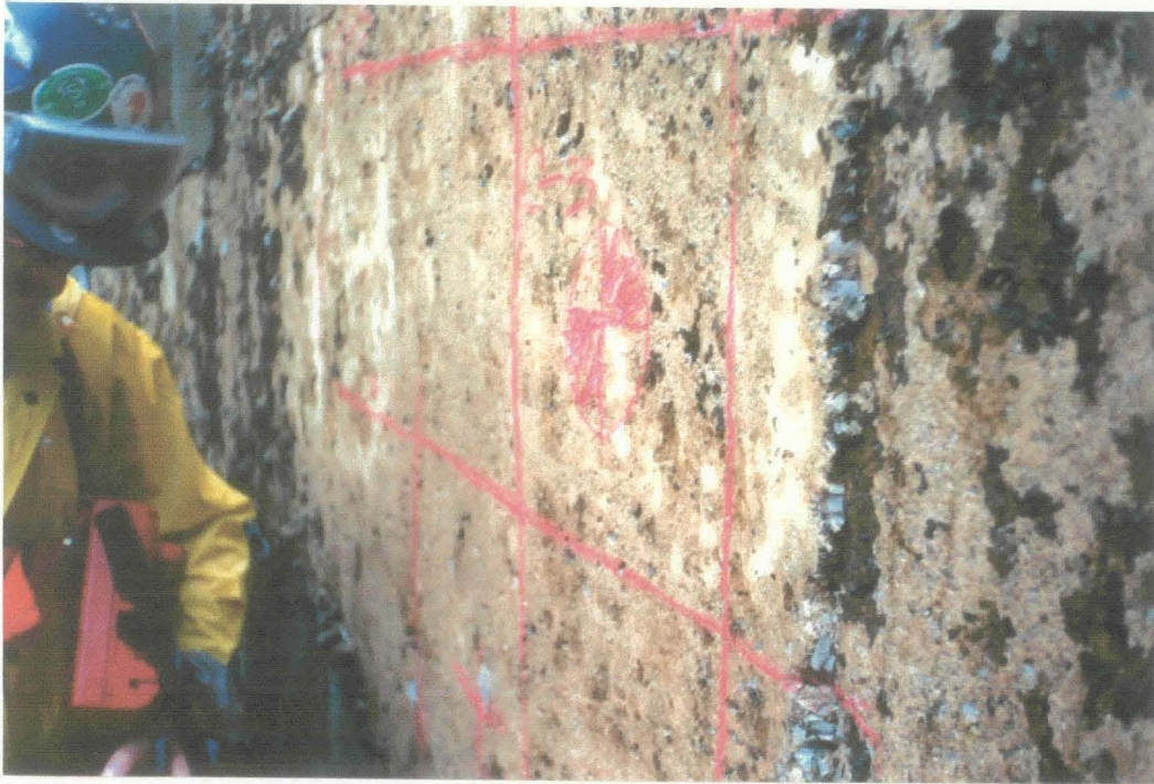
Specimen Photograph No. 15 Core extraction location and reinforcement layout markings
