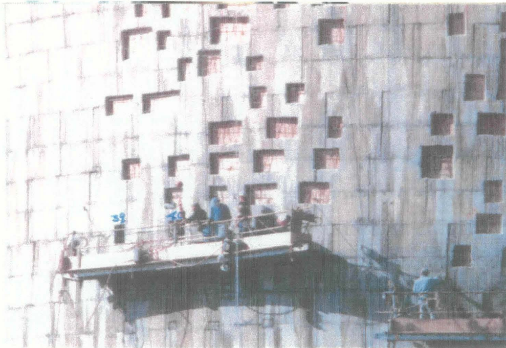
Close-up view of scaffold and formed repair areas
