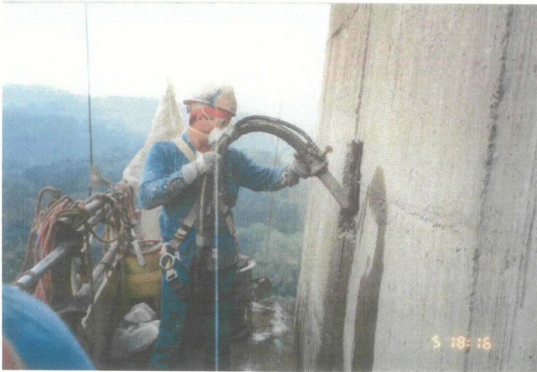
Shotcrete repair in progress
