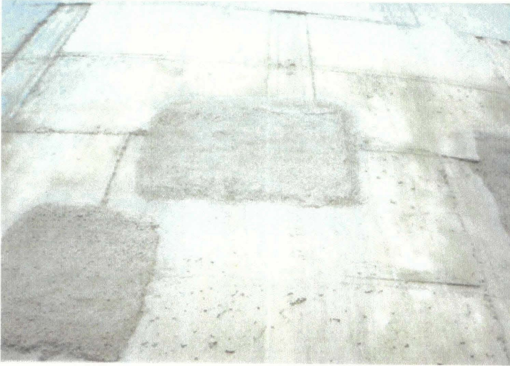
Completed patch repairs
