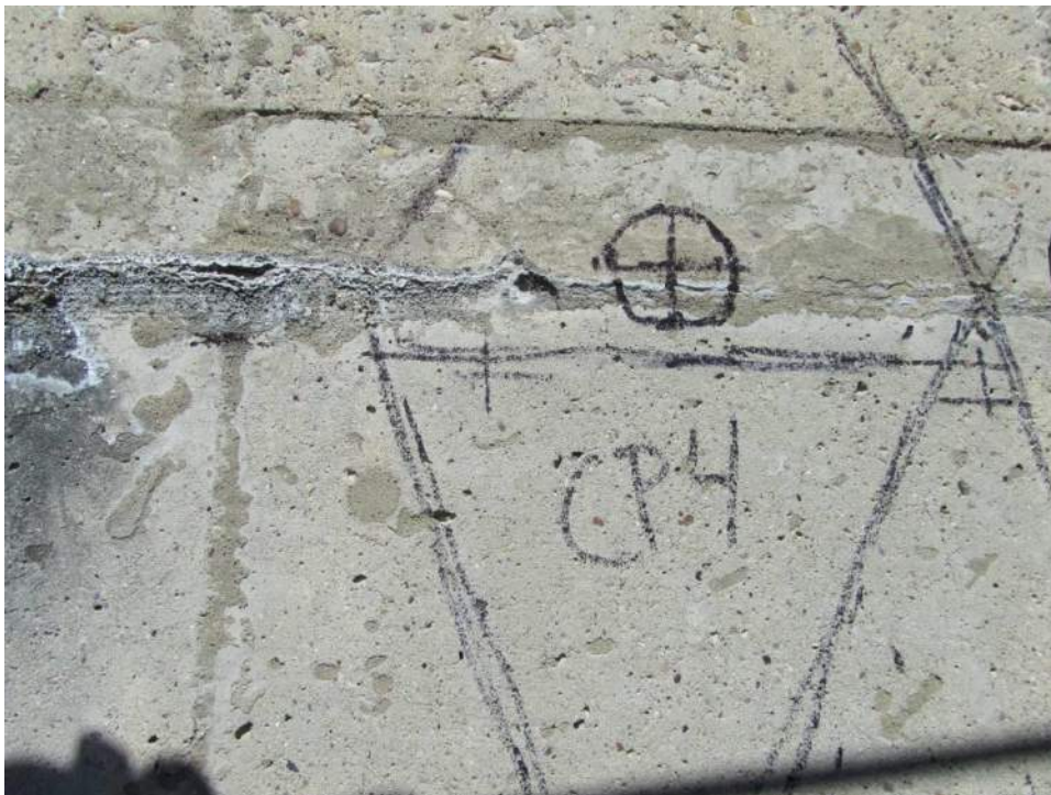
Photo 10. Location marked for a petrography core at a construction joint
