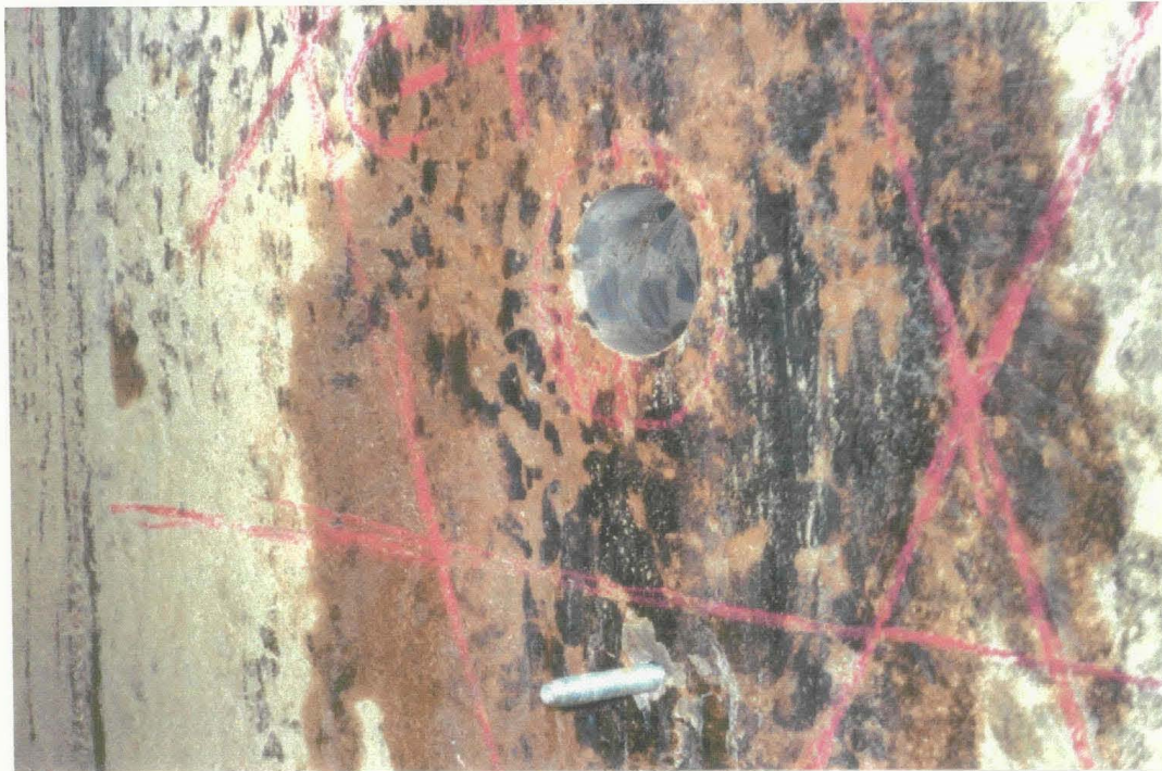
Site Photograph No. 18 Core excavation
