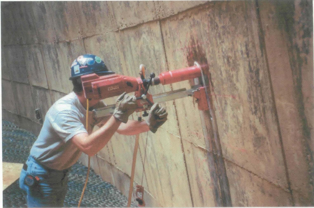
Site Photograph No. 17 Core sample extraction
