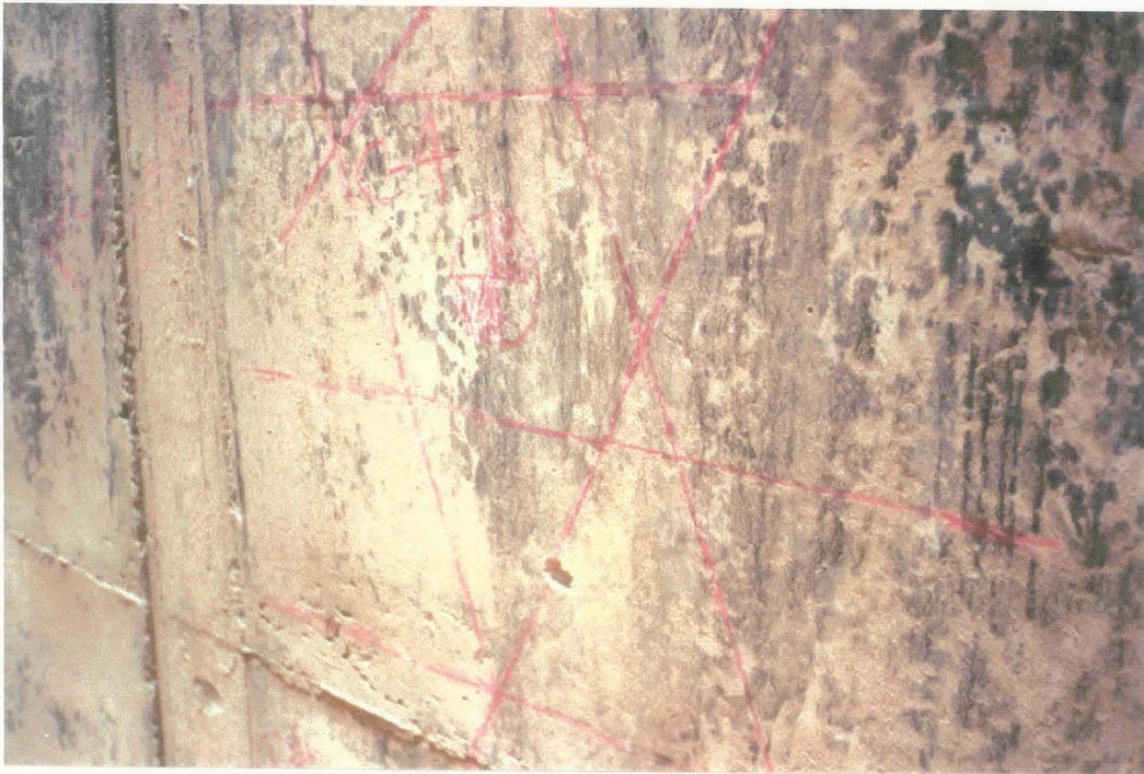
Specimen Photograph No. 16 Core extraction location and reinforcement layout markings
