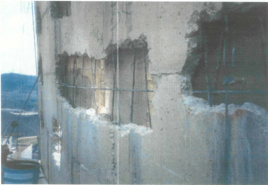
Concrete removal areas with forms
