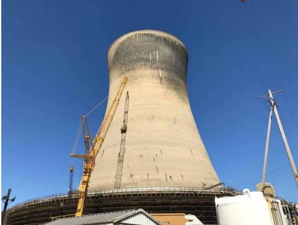
Photo 1. Overview of Unit 2 cooling tower
