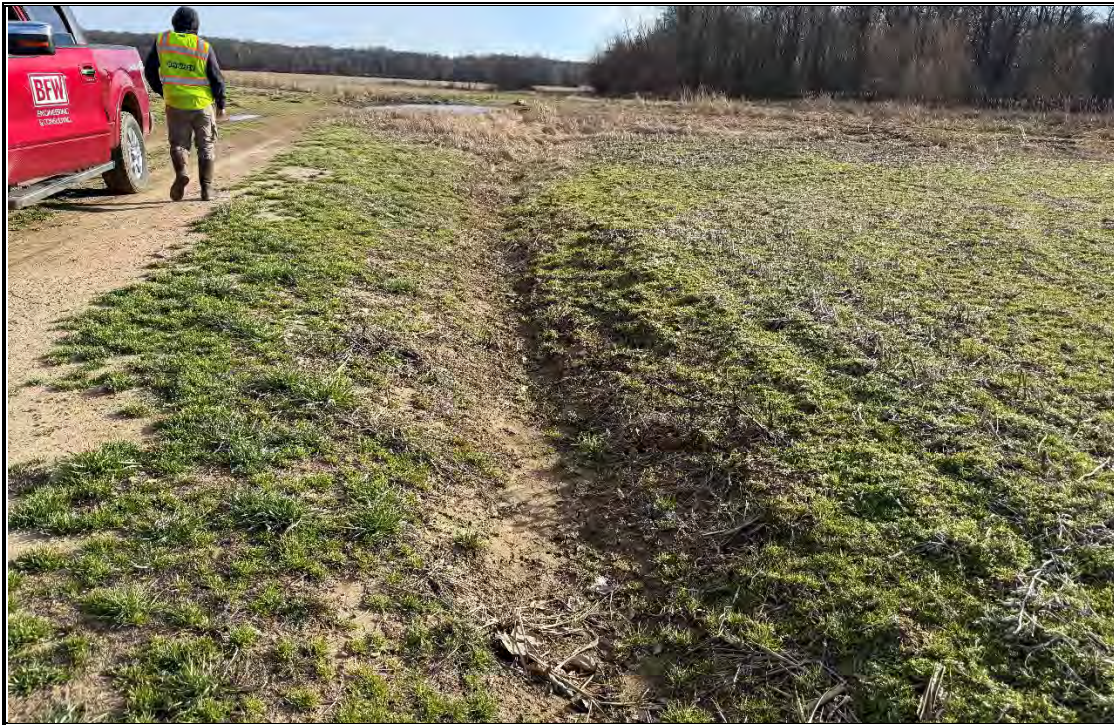
Photograph 7: View of a ditch feature in the central part of the site, facing east from south of Wetland C toward an offsite woodlot. January 13, 2026.
