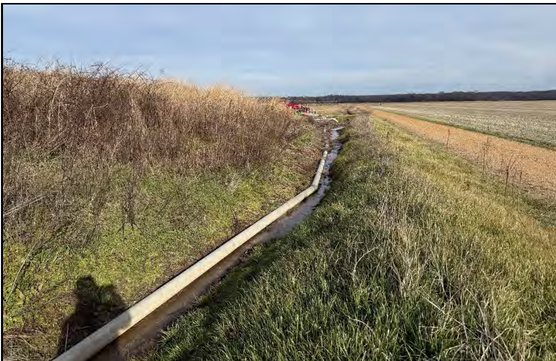
Photograph 14: View of a section of Intermittent Stream C, facing north along the eastern edge of Pond B which is located behind the berm to the left. Irrigation piping is present. January 13, 2026.
