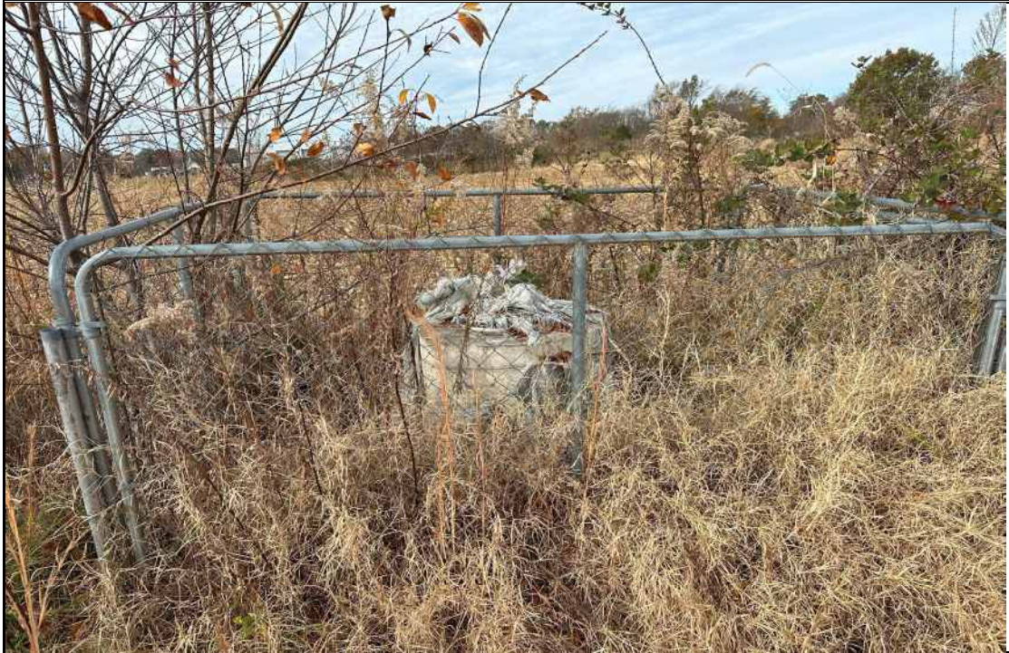
Photograph 51 – Parcel 24 – Concrete well. November 14, 2023
