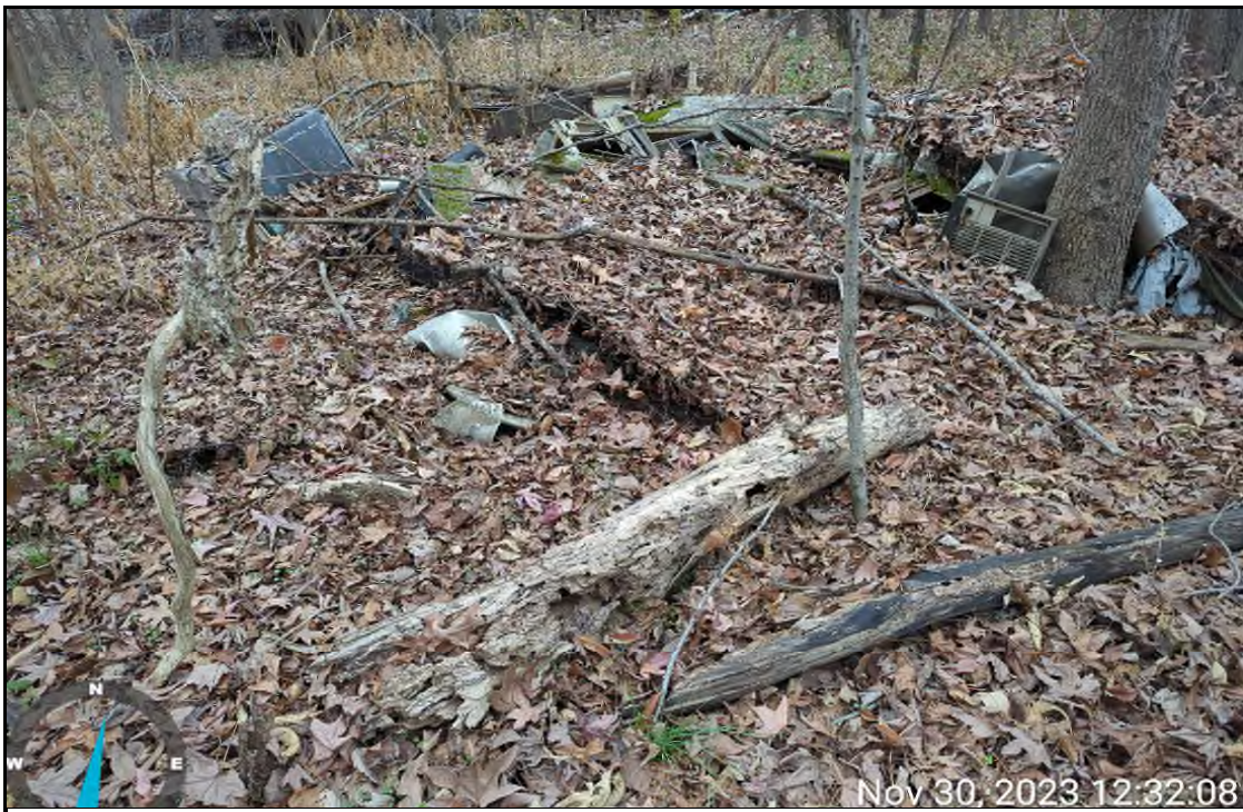
Photograph 24 – Parcel 47 – Collapsed mobile home. November 30, 2023
