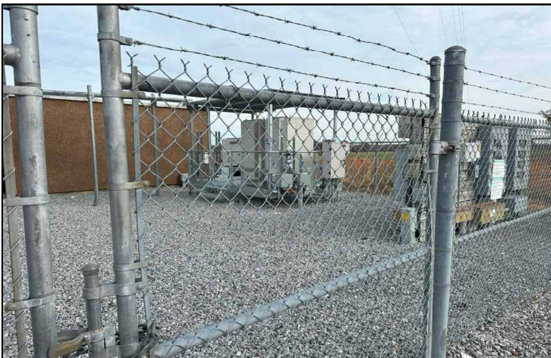
Photograph 50 – Parcel 23 – AT&T power source. November 14, 2023
