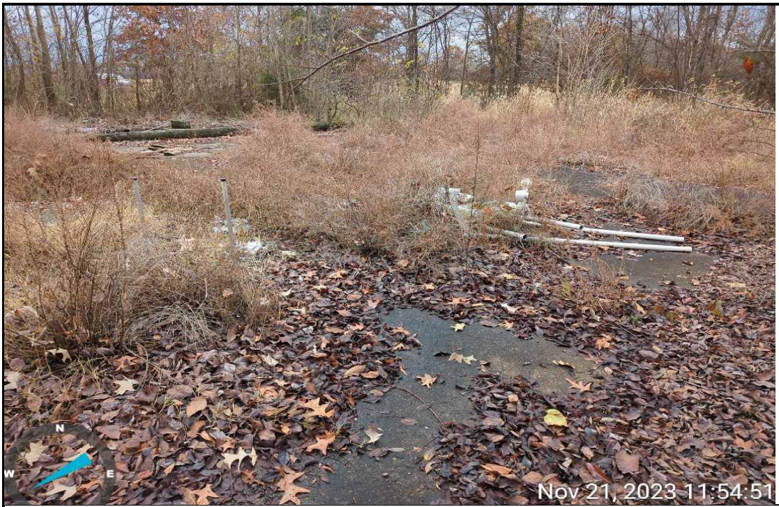
Photograph 32 – Parcel 60 – Concrete foundation. November 21, 2023
