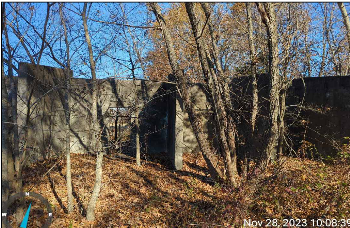
Photograph 26 – Parcel 48 – Concrete building. November 28, 2023
