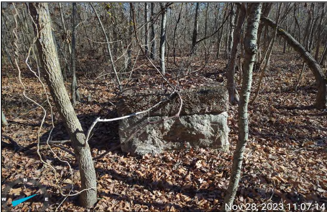
Photograph 27 – Parcel 48 – Concrete structure. November 28, 2023
