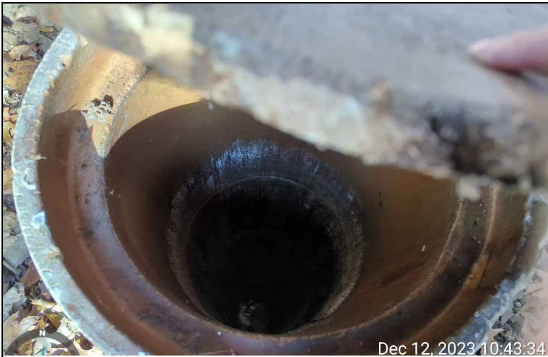
Photograph 43 – Parcel 62 – Concrete well. December 12, 2023
