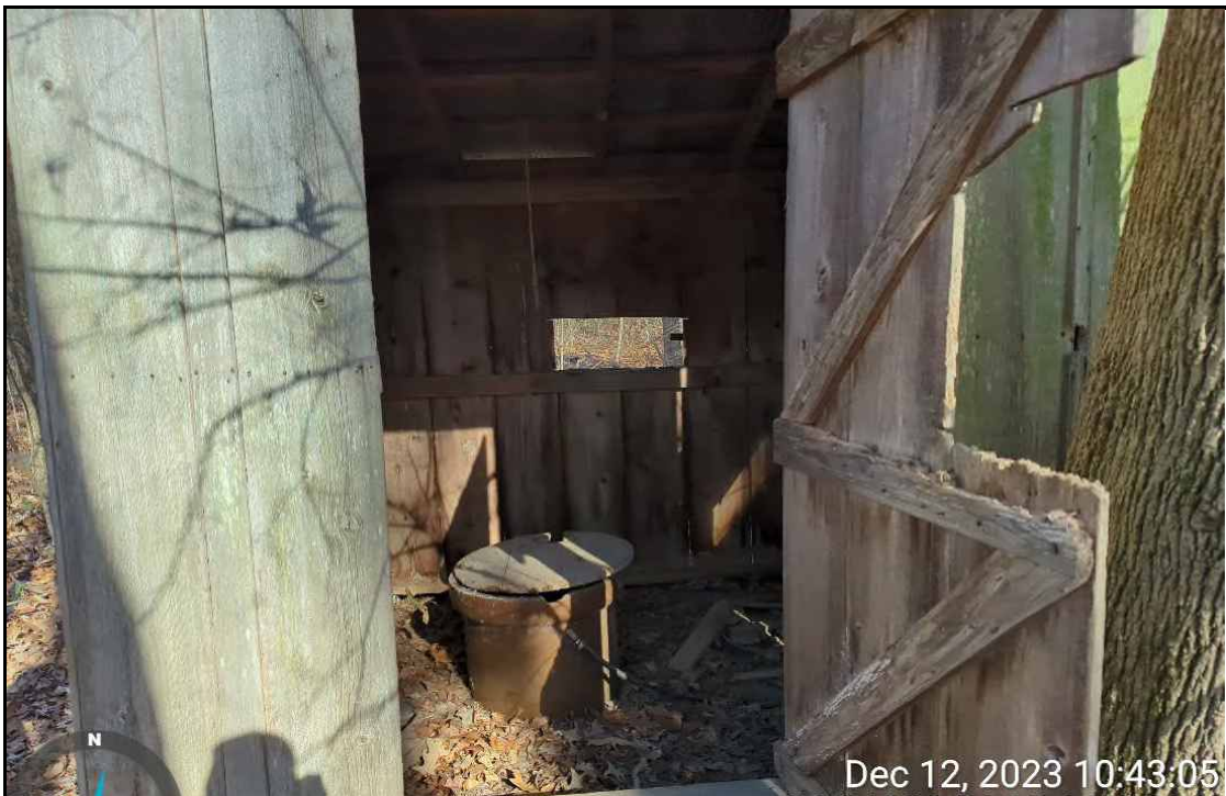
Photograph 42 – Parcel 62 – Old well house. December 12, 2023
