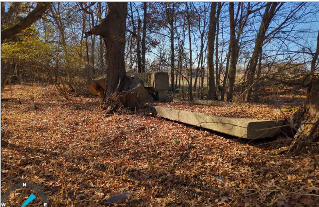
Photograph 21 – Parcel 47 - Concrete foundation. November 28, 2023.
