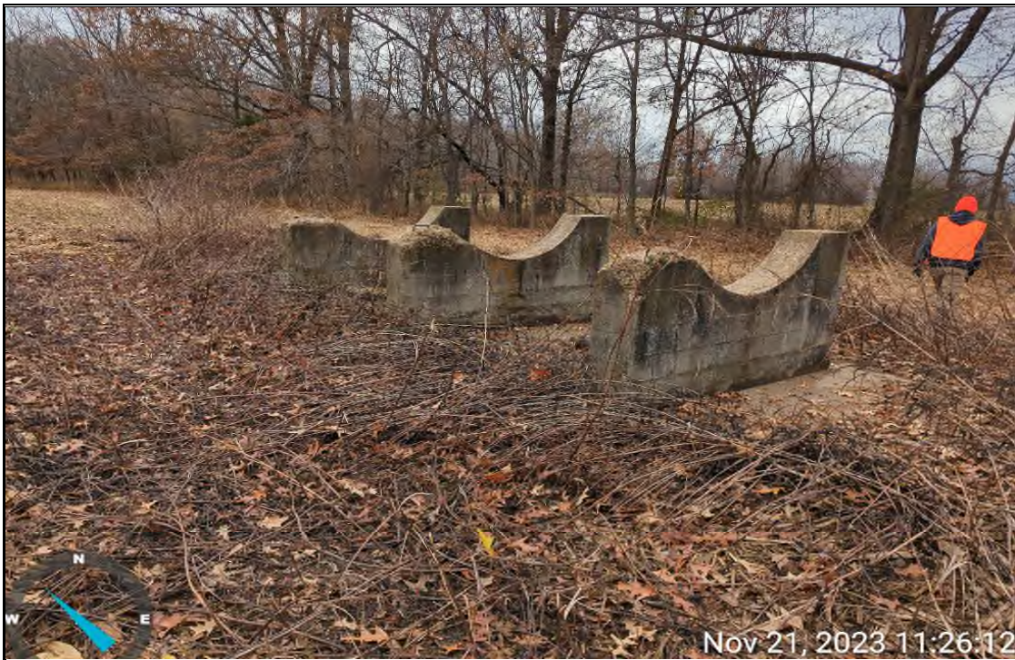
Photograph 29 – Parcel 57 – Aboveground storage tank support. November 21, 2023
