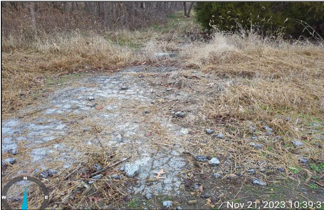
Photograph 33 – Parcel 60 – Concrete foundation. November 21, 2023
