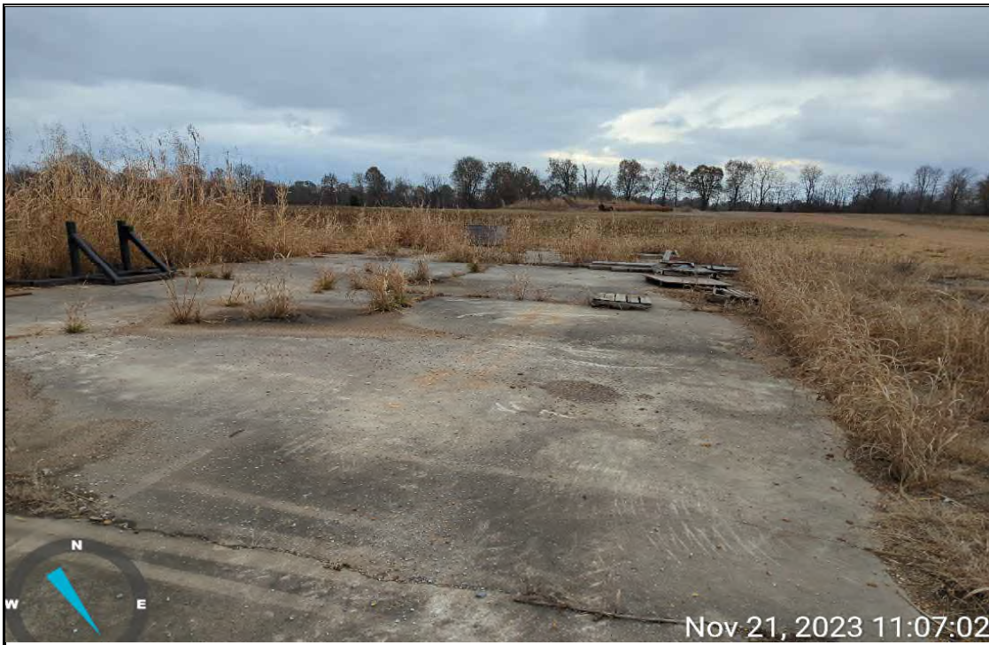
Photograph 31 – Parcel 60 – Concrete foundation. November 21, 2023
