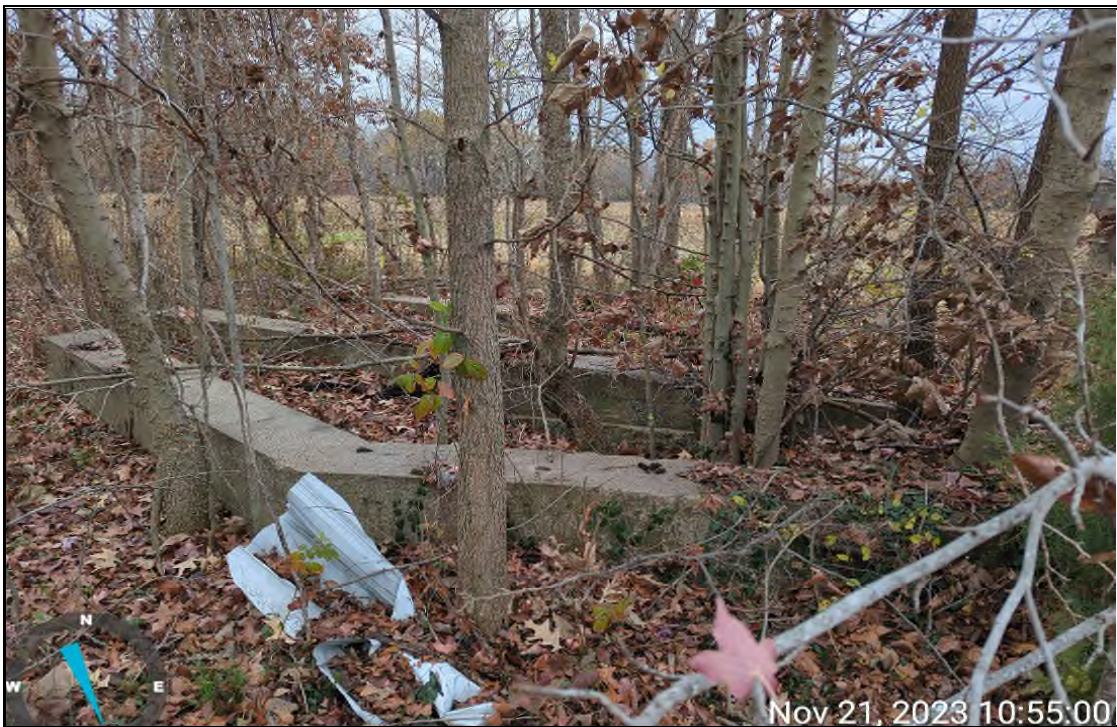
Photograph 41 – Parcel 61 – Concrete foundation. November 21, 2023
