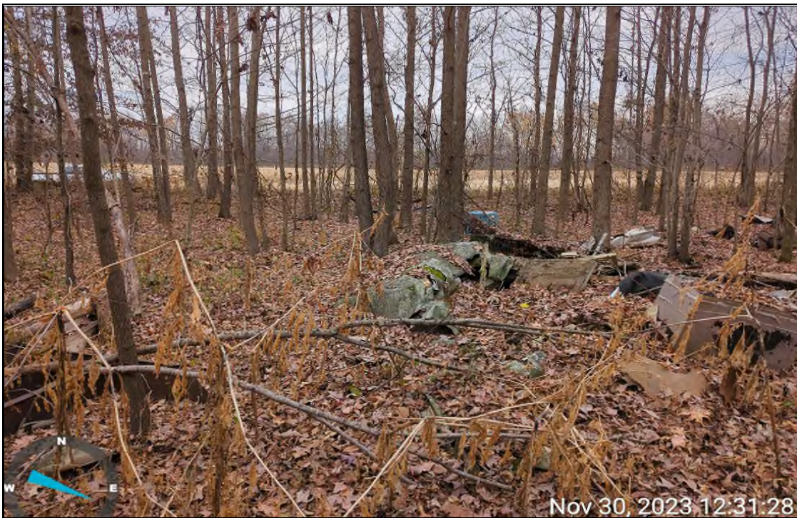
Photograph 23 – Parcel 47 – Collapsed mobile home. November 30, 2023
