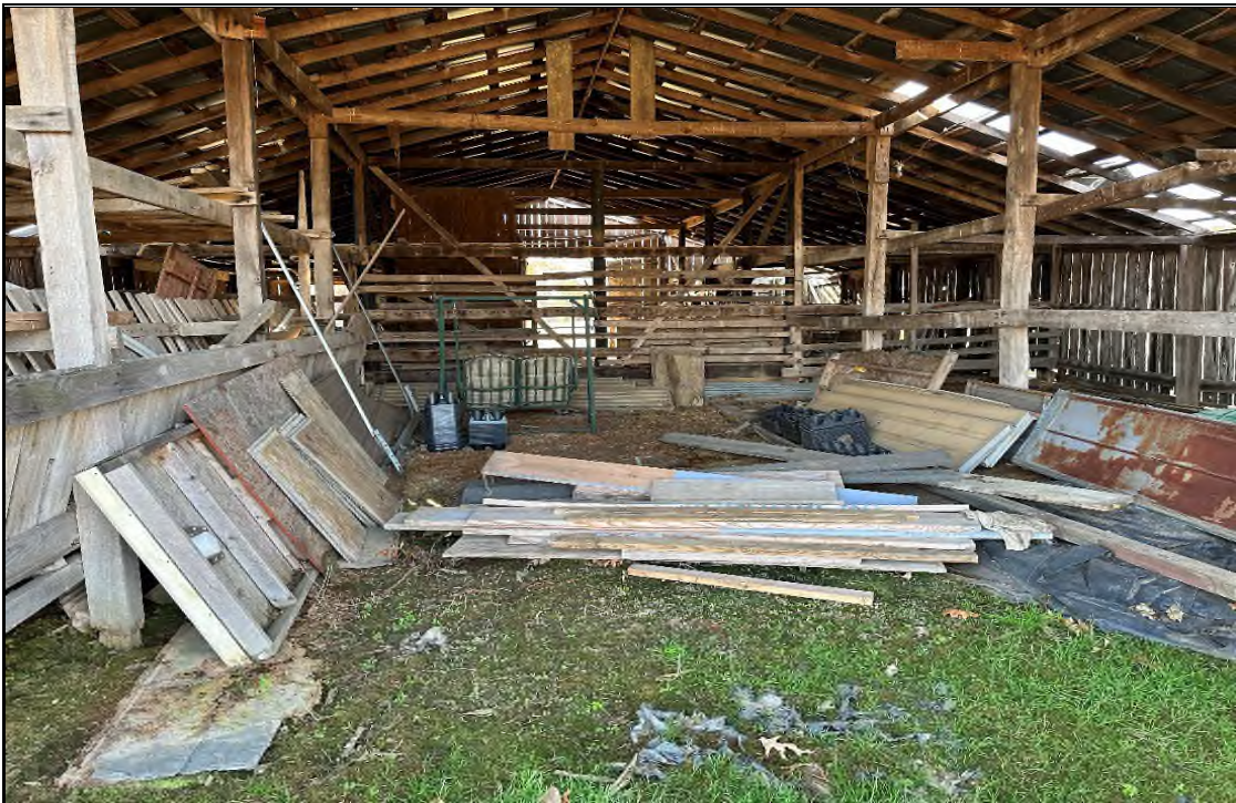
Photograph 12 – Parcel 36 – Inside of old barn. November 13, 2023.
