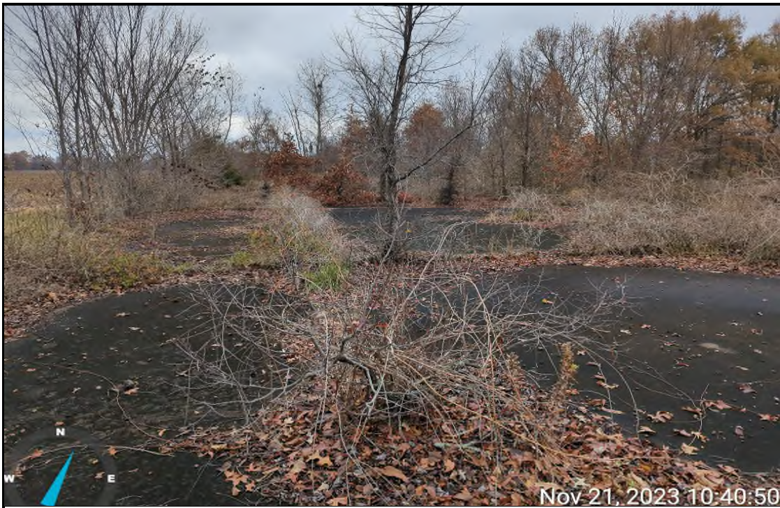
Photograph 40 – Parcel 61 – Concrete foundation. November 21, 2023
