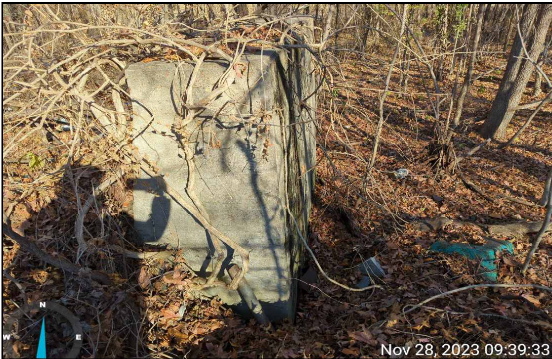
Photograph 46 – Parcel 67 – Concrete wall. November 28, 2023
