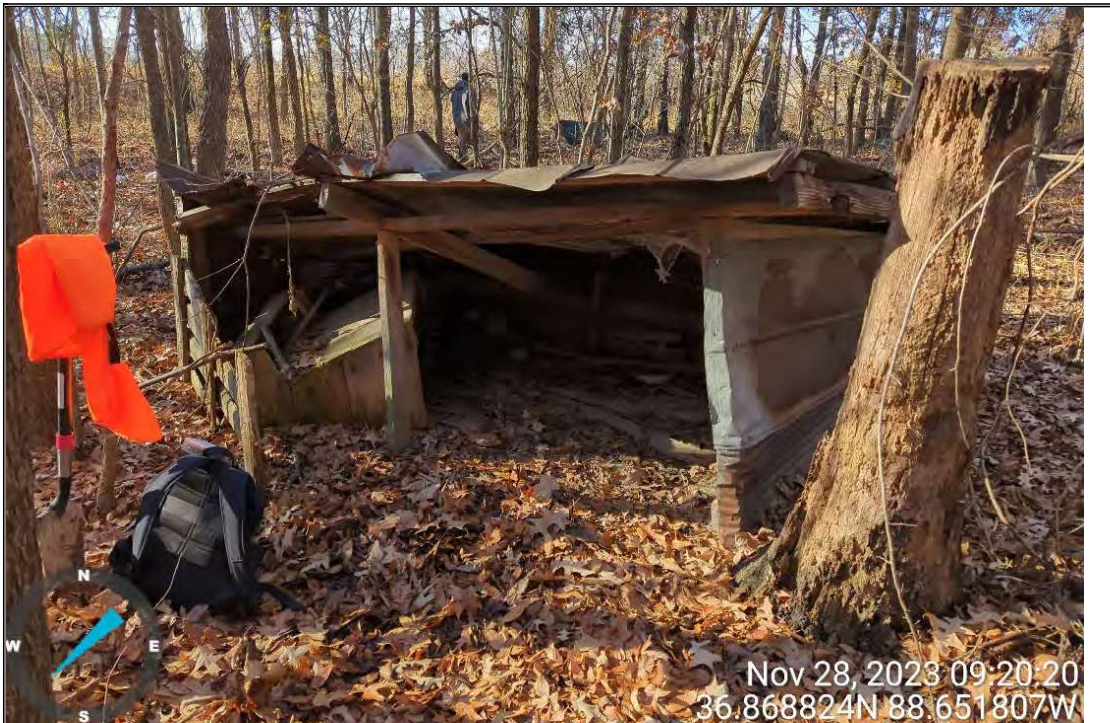
Photograph 28: A few abandoned small outbuildings are present within the study area. This shed on Parcel 60 is a typical example. November 28, 2023.
