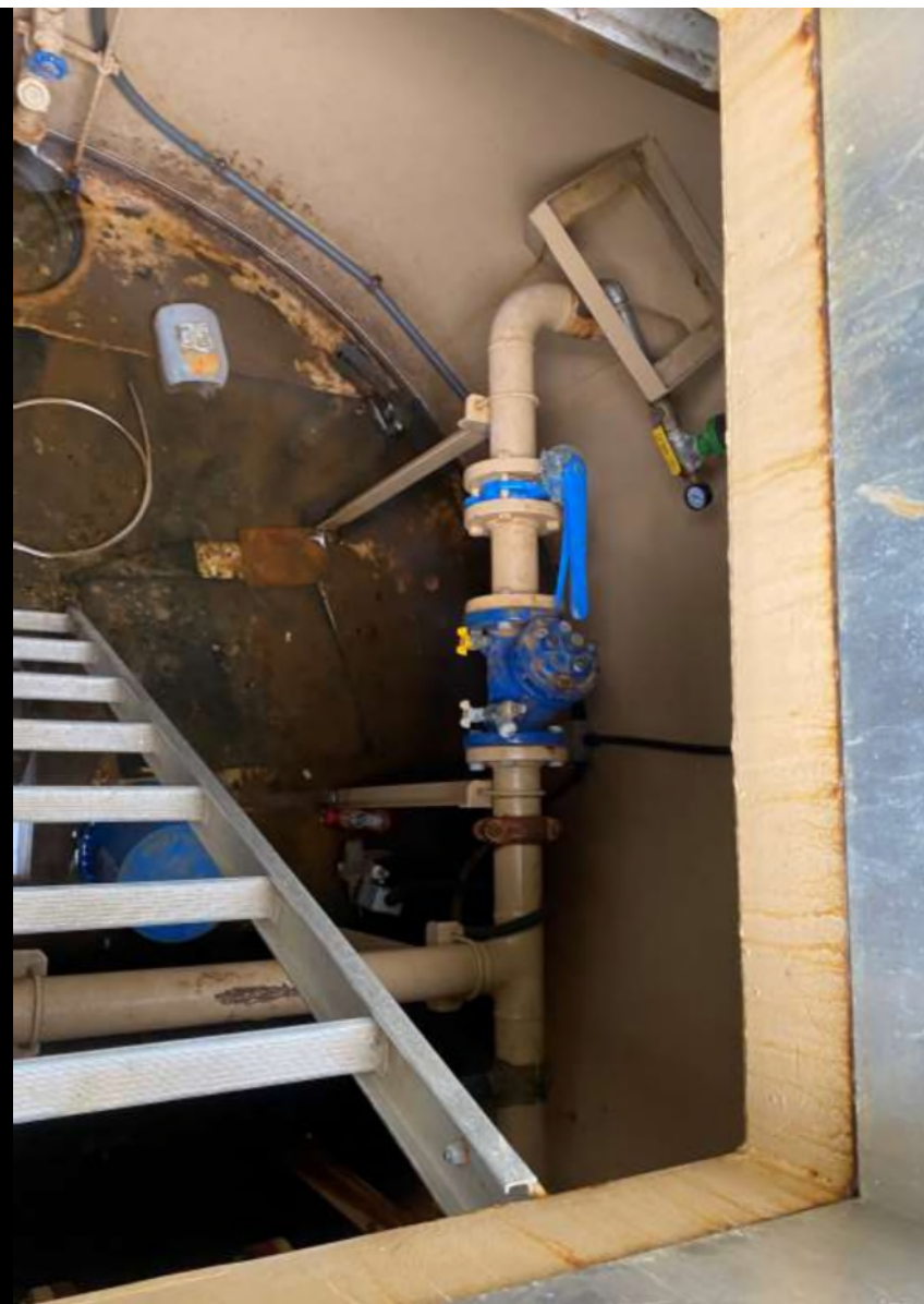
interior of the Wood Creek master meter pit
