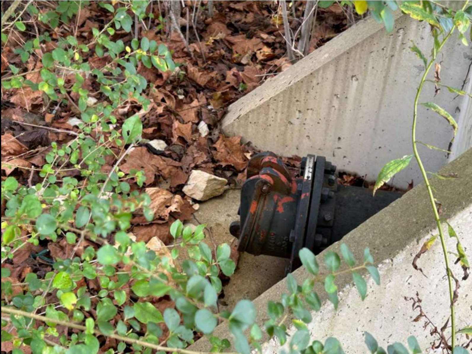
tank overflow outlet
