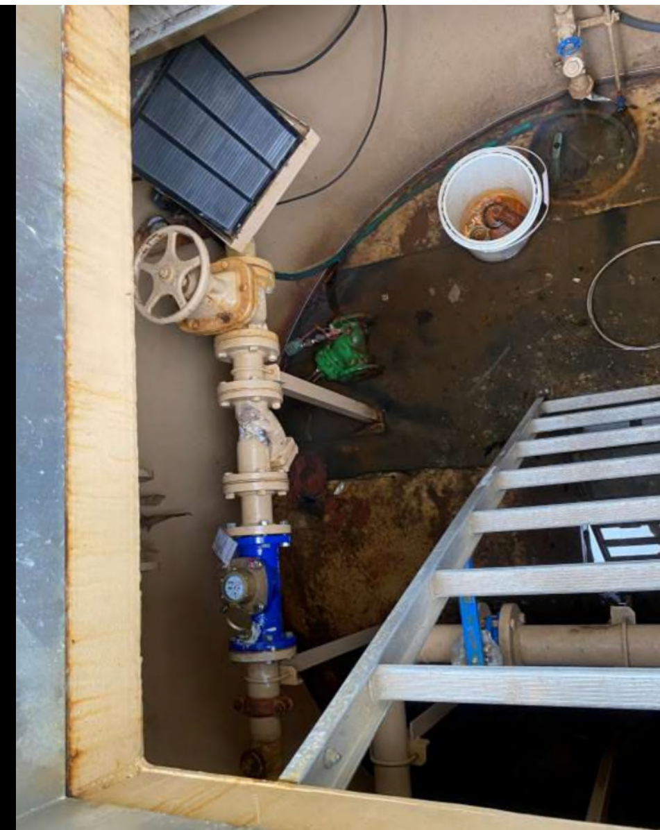
interior of the Wood Creek master meter pit
