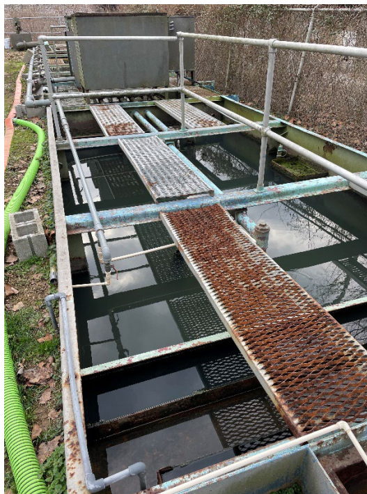
Caption: WWTP clarification chamber
