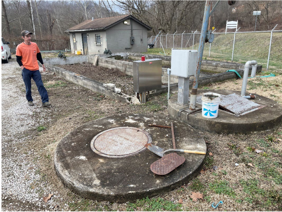
Caption: WWTP Influent pump station wet well
