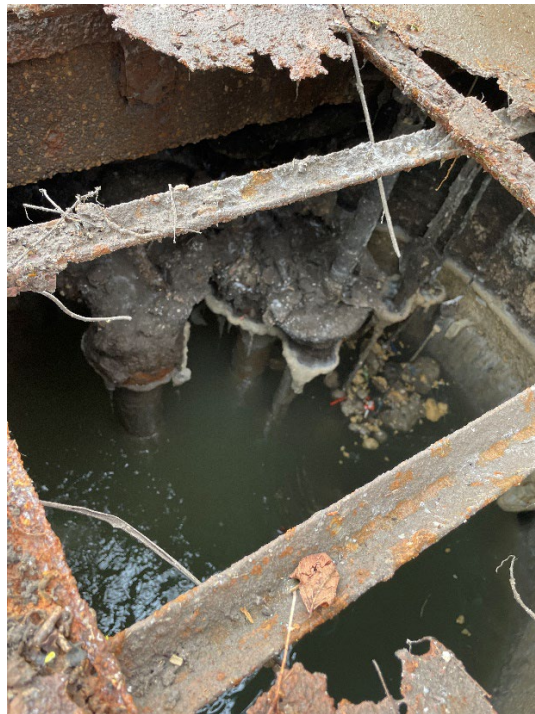
Photo #10 Caption: Wastewater lift station wet well
