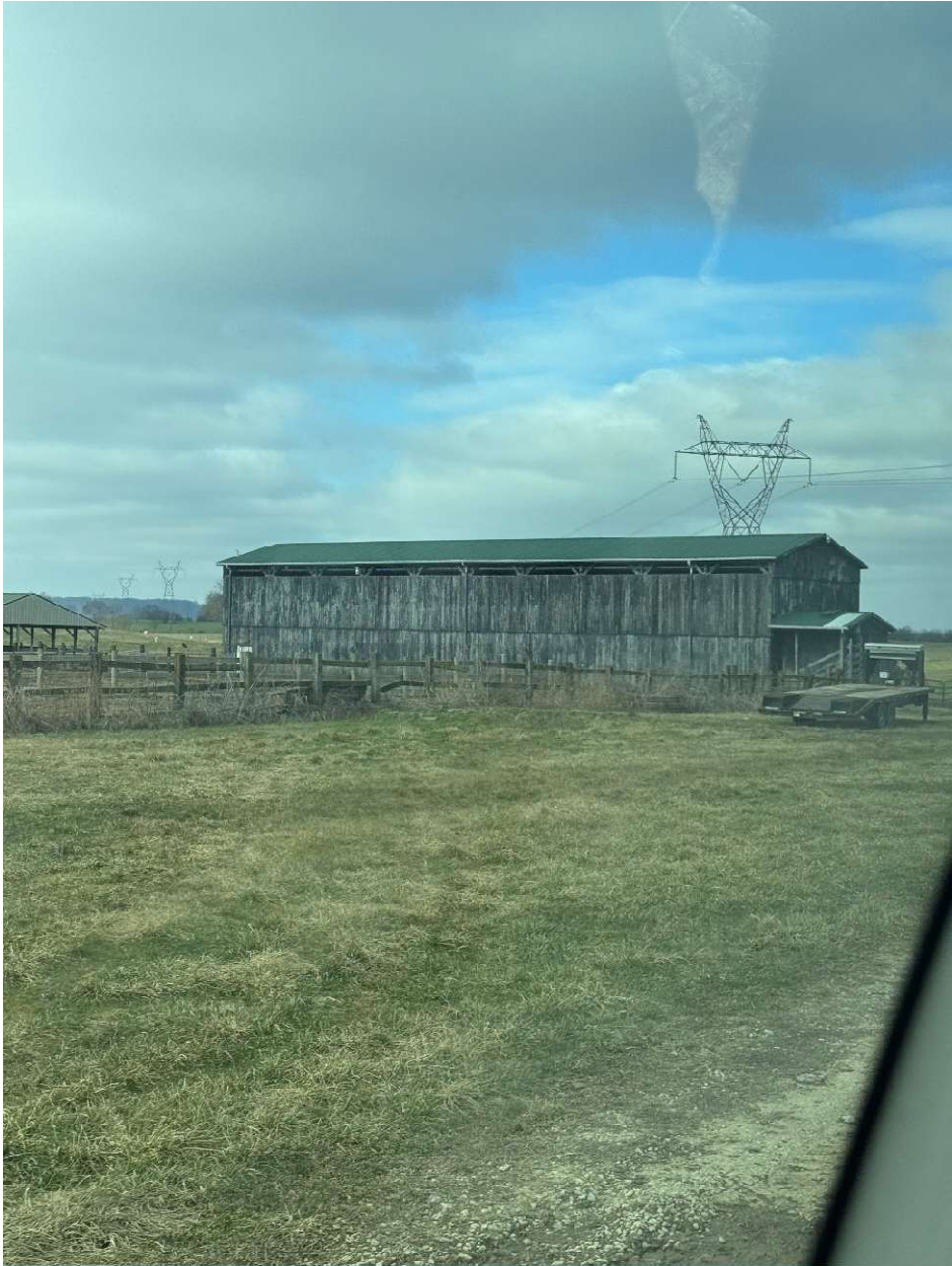
Figure 4 - Stop 1 – View 2, Barn within Project Boundary by Southeast Entrance
