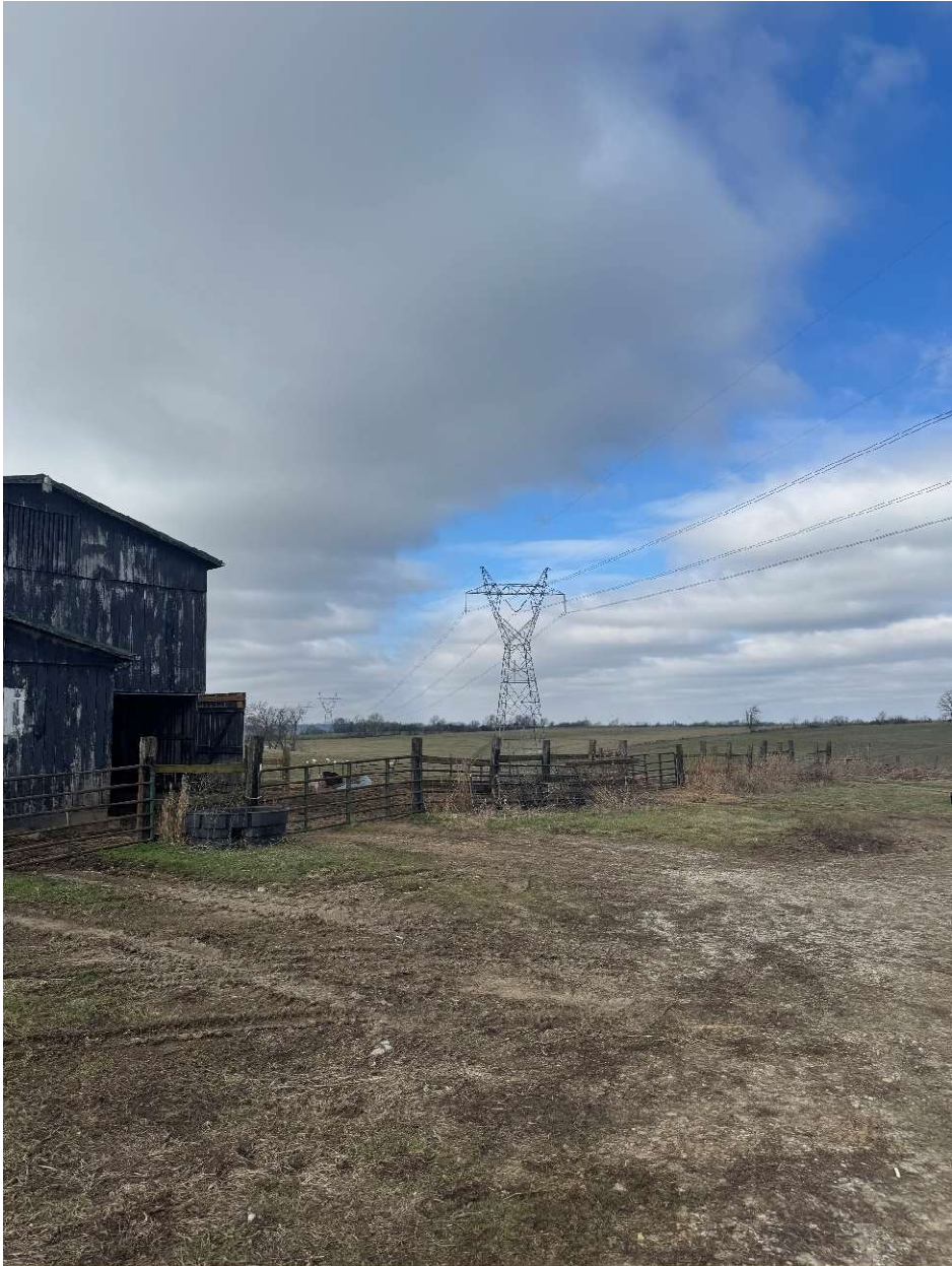
Figure 12 - Stop 1 – View 6, Hardin County to Brown North (KU) 345 kV transmission line 1
