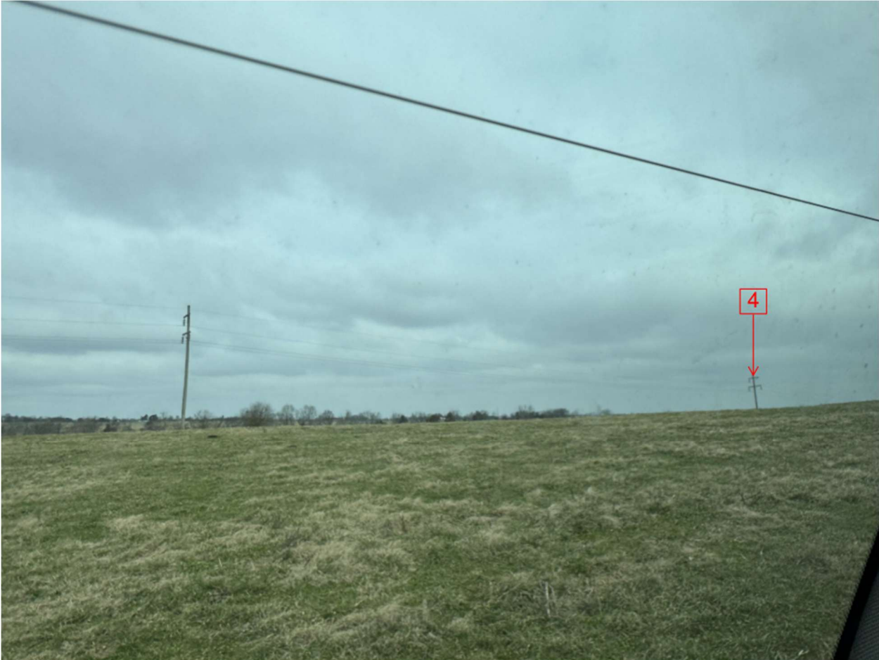
Figure 37 - Stop 3 – View 4, Sulphur Creek to Loretto 69kV EKP pole 4
