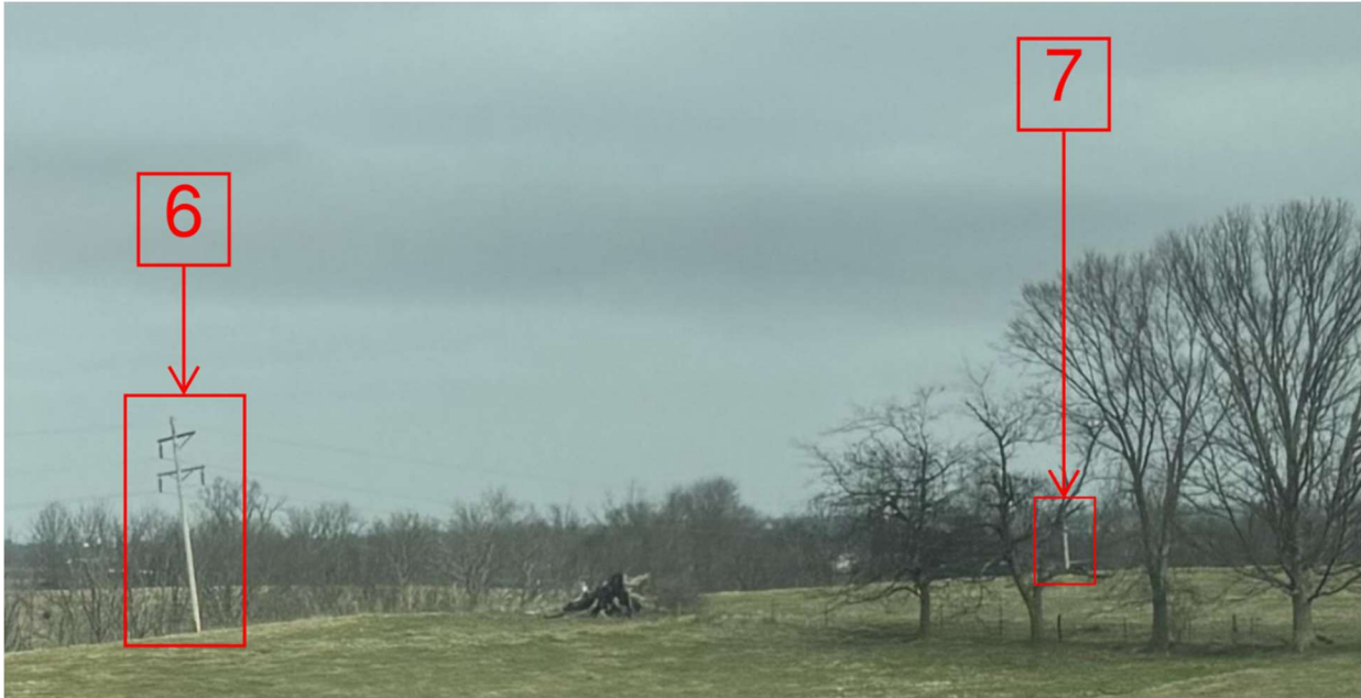
Figure 42 - Stop 4- View 2 B, Sulphur Creek to Loretto 69kV EKP poles 6&7
