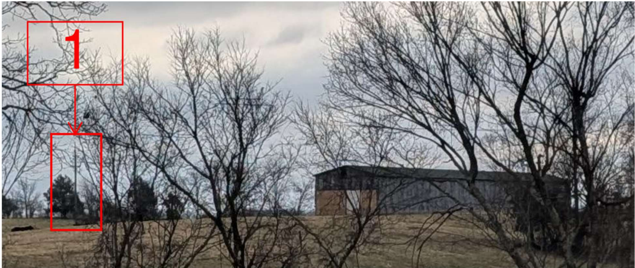
Figure 31 - Stop 3 – View 1 B, Sulphur Creek to Loretto 69kV EKP pole 1
