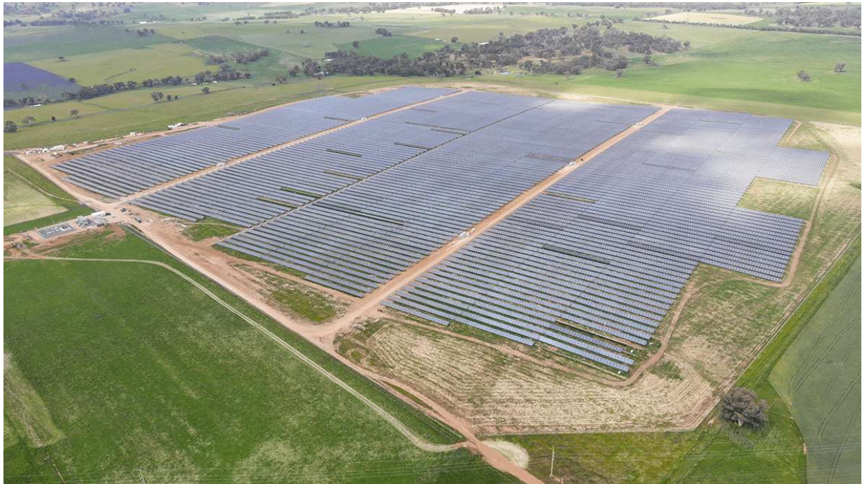
Picture (3) Solar Modules Installed on Farmland 3
