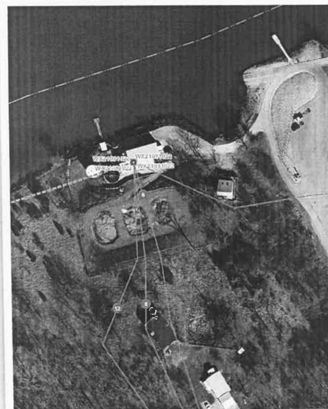
Bullock Pen Water Treatment Plant
