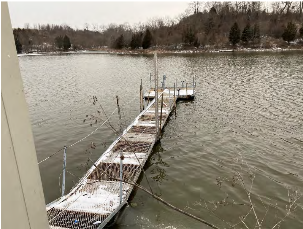
Walkway to Raw Water Intake
