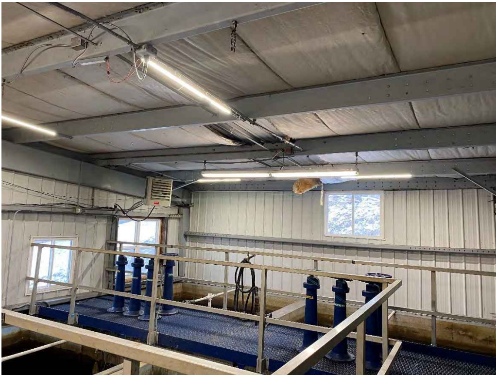
Walkway Above Filter Basins
