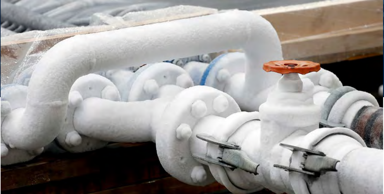
Frozen pipelines during Winter Storm Elliott caused difficulties starting the gas units.
