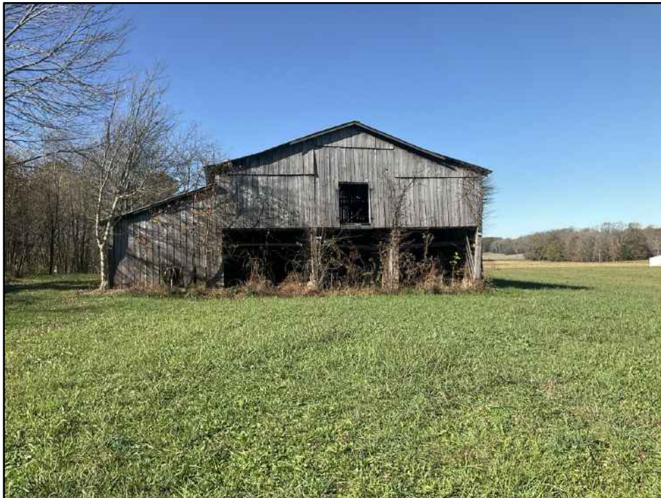
Photograph C-14: Barn at site 15Gn86; facing west.
