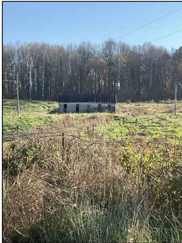
Photograph C-24: Structure at site 15Gn91; facing south.
