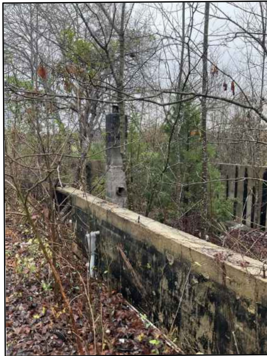
Photograph C-29: Overview of house foundation at site 15Gn96; facing north.
