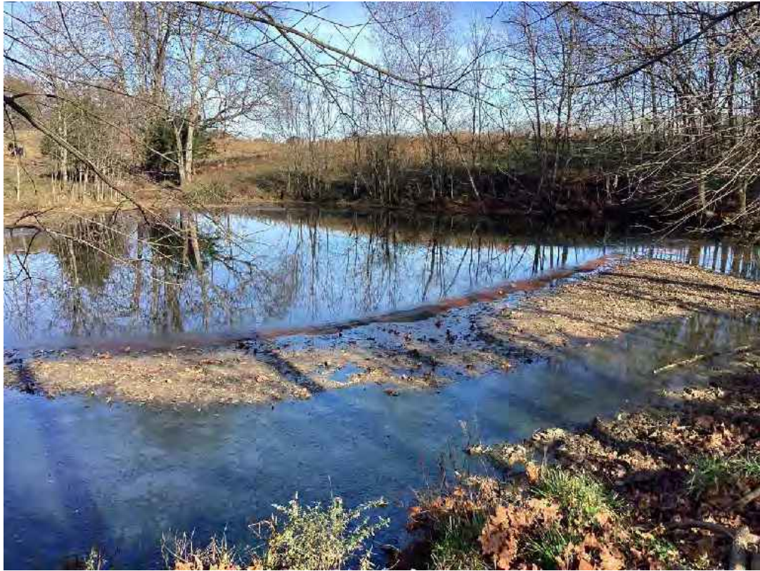
Photo C-139: View of PA27, facing northeast.
