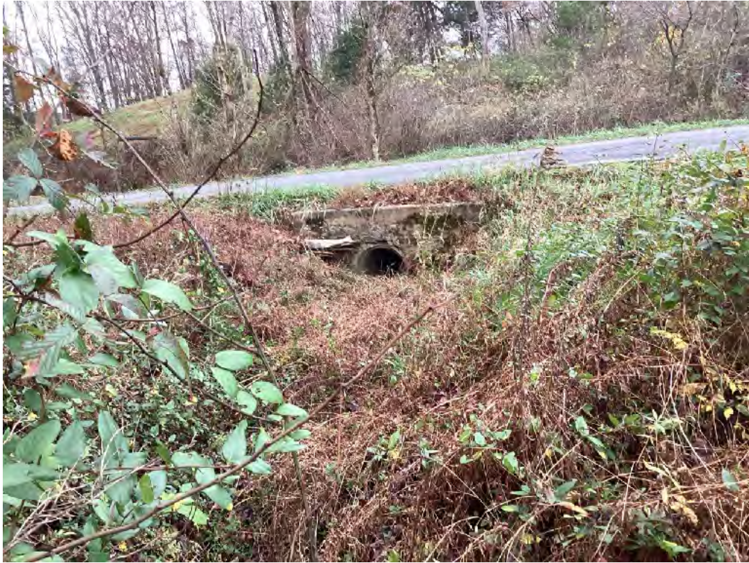
Photo C-80: View of ephemeral SA43, facing south.
