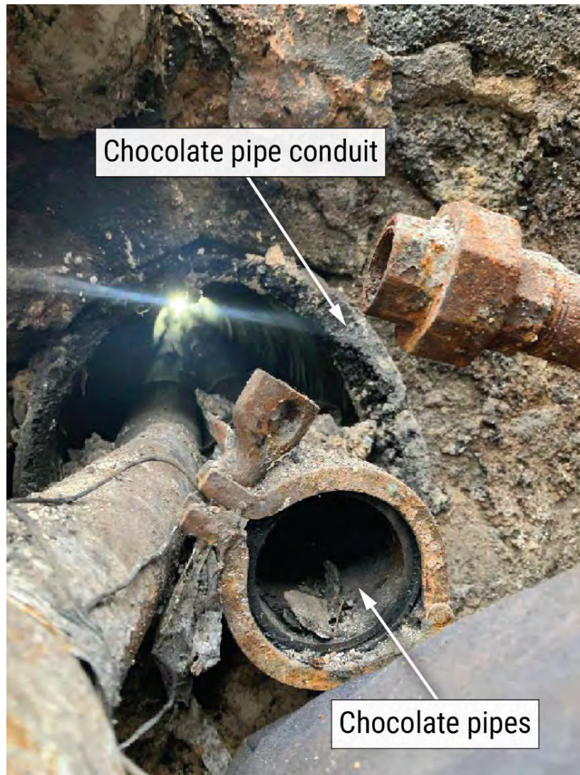
Figure 12. A view of one of the chocolate pipe conduits from the Building 2 basement.
