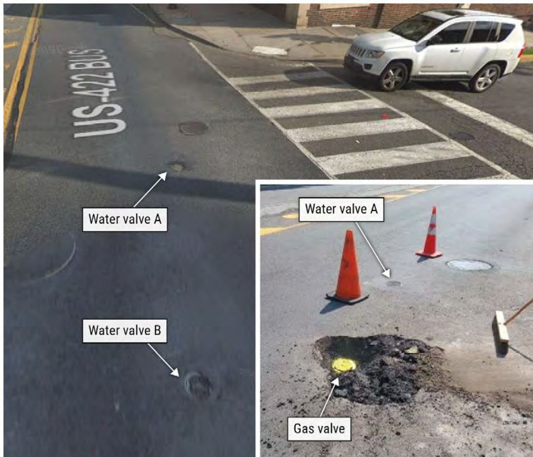
Figure 8. South 2nd Avenue and Penn Avenue intersection in 2018 ( main image ) and during an excavation in 2024 ( inset ); water valve A had a gas cover. (Source: Google Street view via UGI.)
