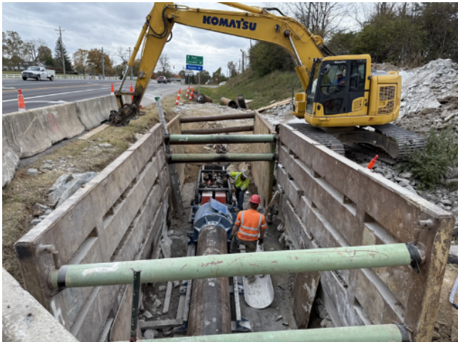
9 Jack-and-bore (left) and open-trench (right) pipe installations for the Millersburg Transmission Main Project
