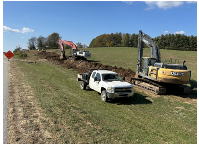
9 Jack-and-bore (left) and open-trench (right) pipe installations for the Millersburg Transmission Main Project
