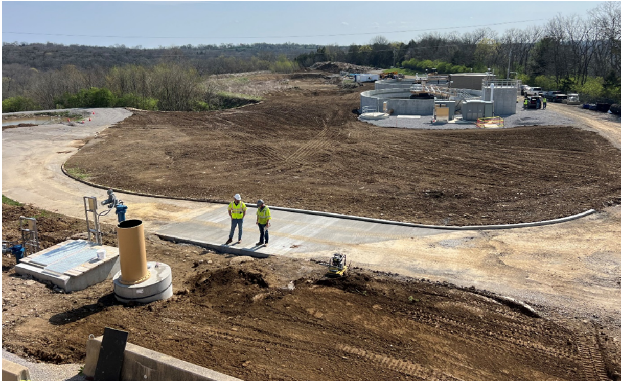
KRS1 Gravity Thickeners Project, including the two 70' diameter concrete tanks
