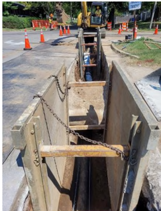
Water main installation for the New Circle Widening Main Relocations Project
