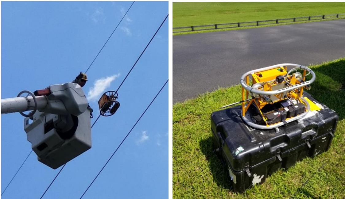
Figure 6-1 Non-destructive Testing of Overhead Conductor
