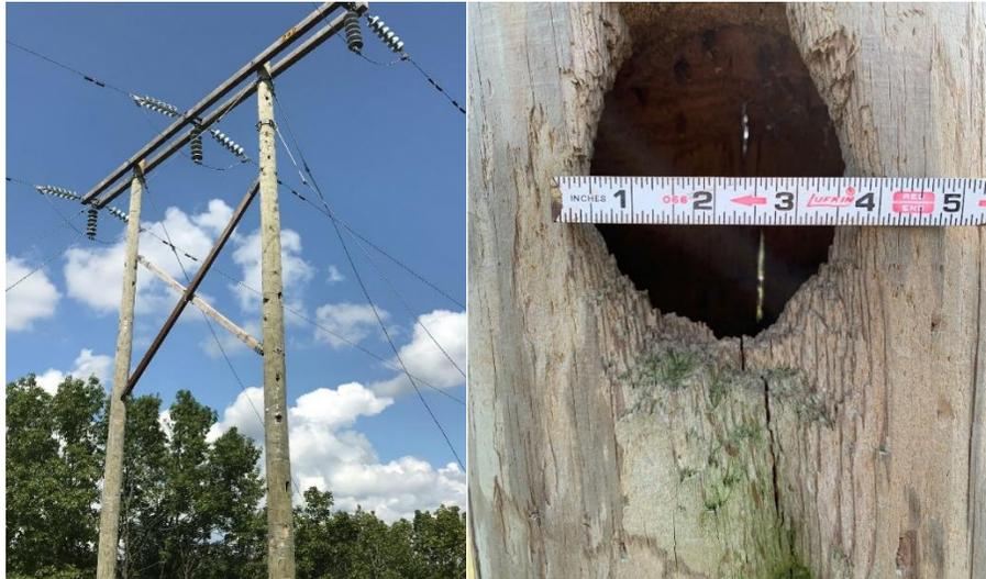
Figure 2-7 Woodpecker Damage to Wood Structure
