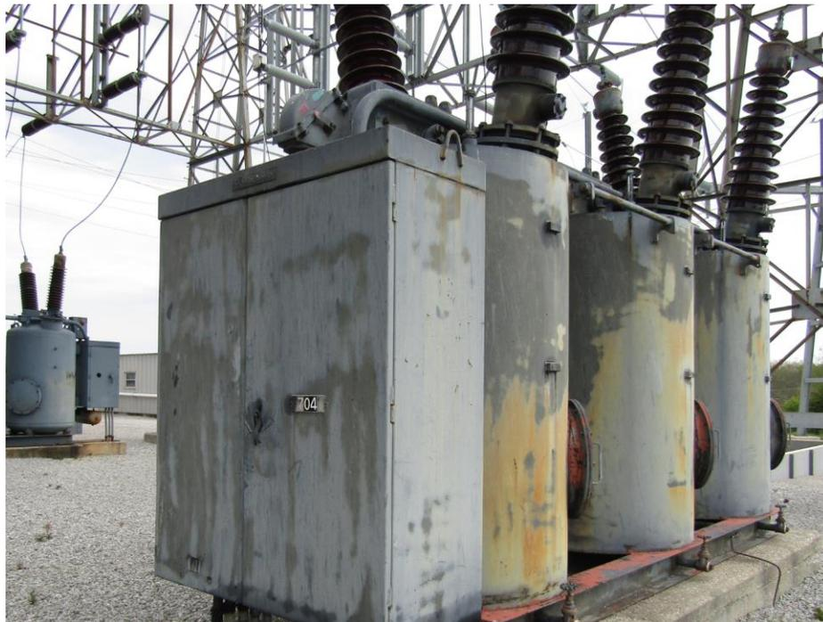
Figure 2-8 Aged 138kV Oil Circuit Breaker
